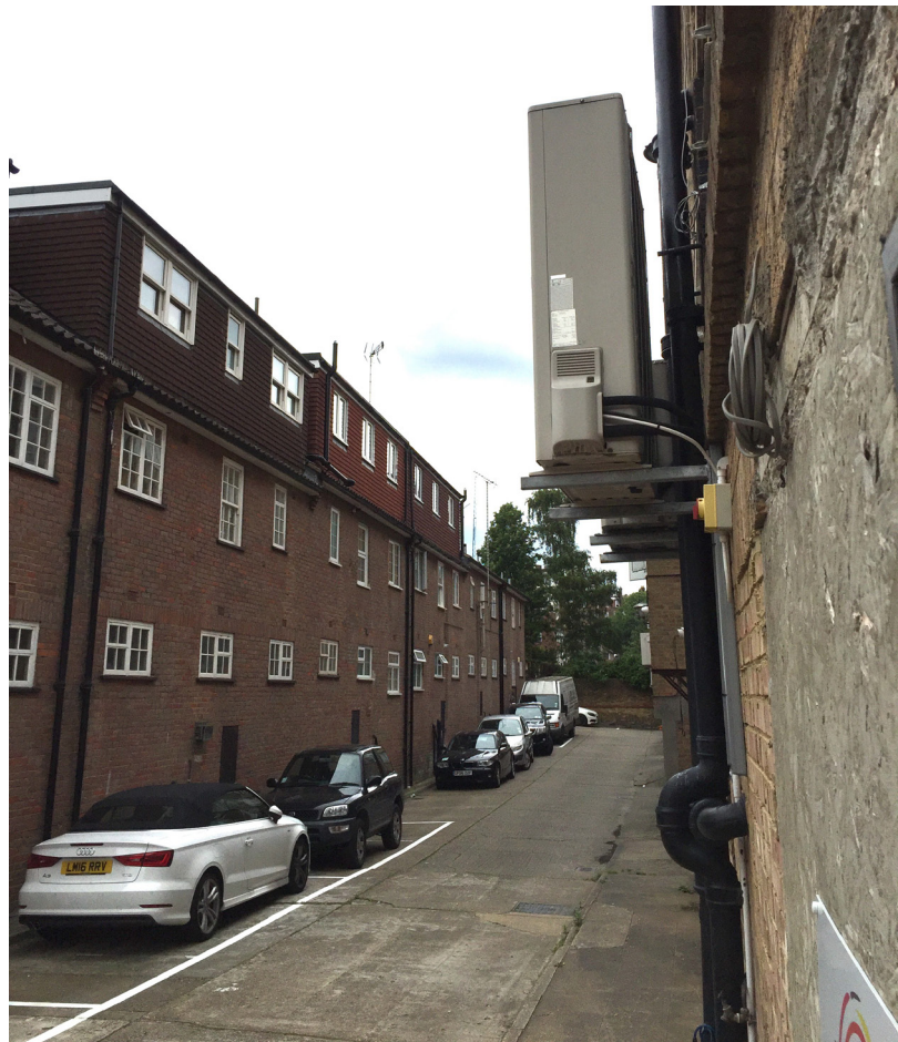
looking north along rear of 16-26 Fairfax Place facing onto private service road
