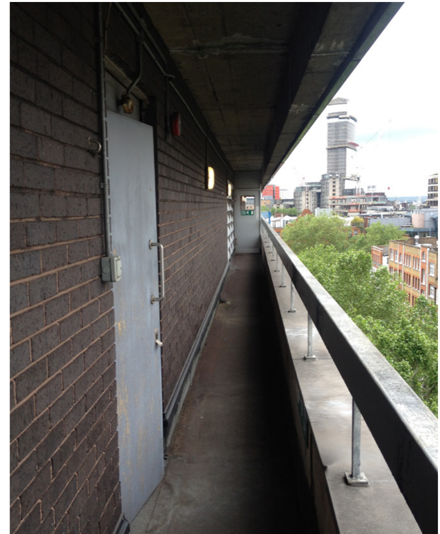
3- Existing entrance door to Terrace
