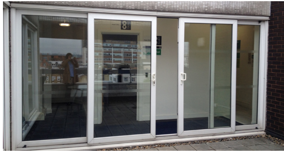
Existing doors ( to be demolished )
