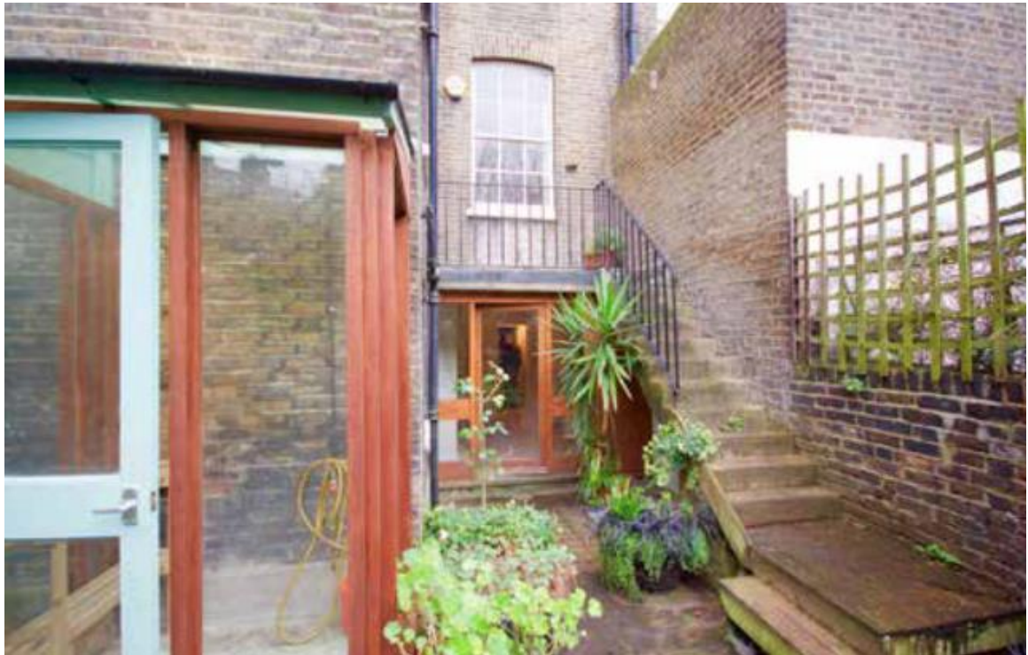
3. Existing glazed lean-to
