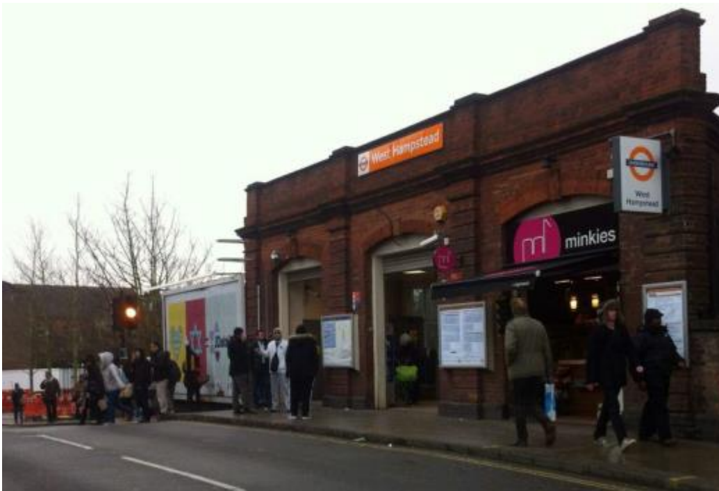
Figure 1: Existing West Hampstead narrow entrance
