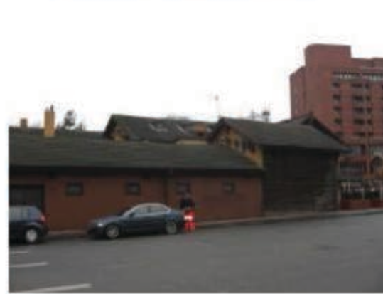
5 Avenue Road elevation
