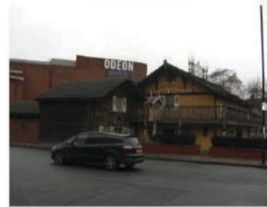
6 Avenue Road elevation
