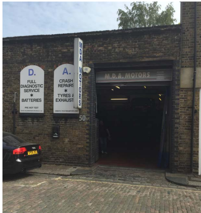
Figure 6: Front elevation of property
