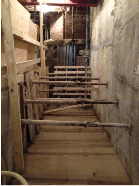
Figure 5 Example of completed walls and back propping to central soil mass
