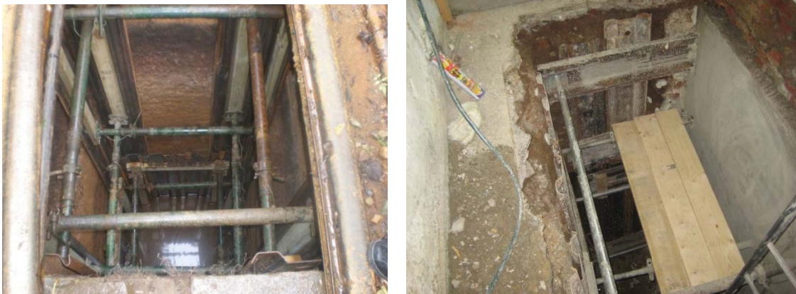
Figure 3 Propping examples
