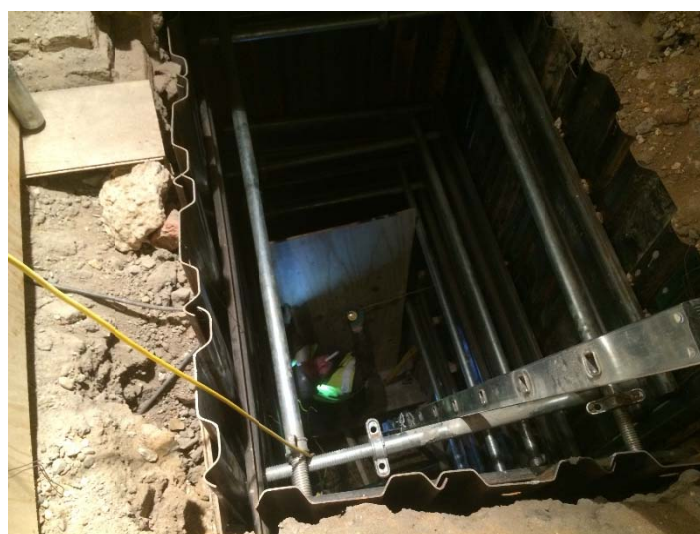
Figure 4 Examples of excavations of pins
