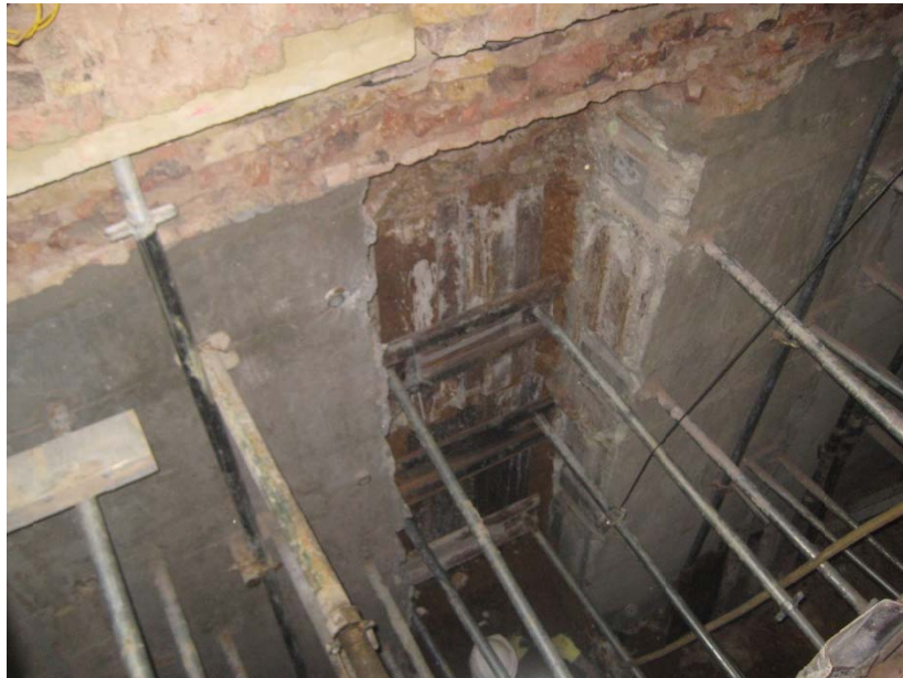
Figure 6 Example of trench sheet back propping
