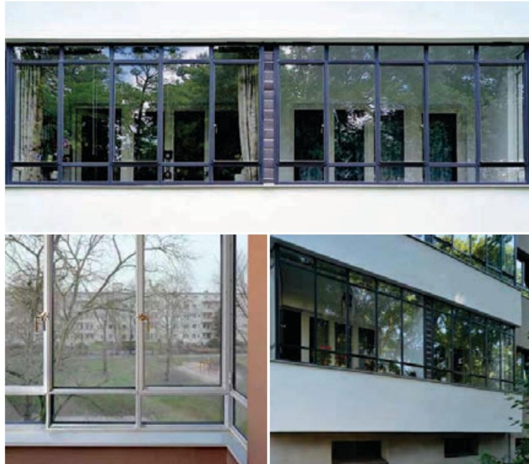
During the restoration work of this district, which has recently started, the replacement of doors and windows has been the object of a specific evaluation by the designers. The old iron windows needed to be replaced with new window systems that could guarantee not only living comfort, but also the preservation of the previous design and size while guaranteeing, at the same
