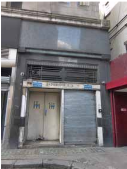
34. Section of the original shop front/entrance to Bainbridge Street, 2015 (DIA).
