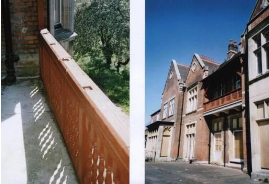
MMP15, 16 Original First Floor balcony balustrade on West Elevation
