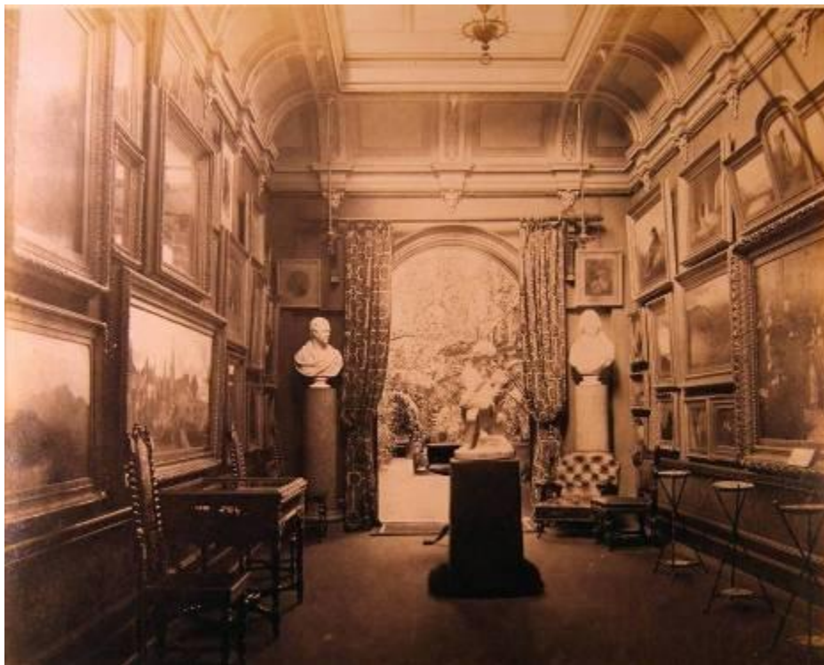
MMJ13 080179/14 shows the same room looking north into the Conservatory. The arch itself is exposed on the north elevation, following demolition of the later extensions for the hospital use.
