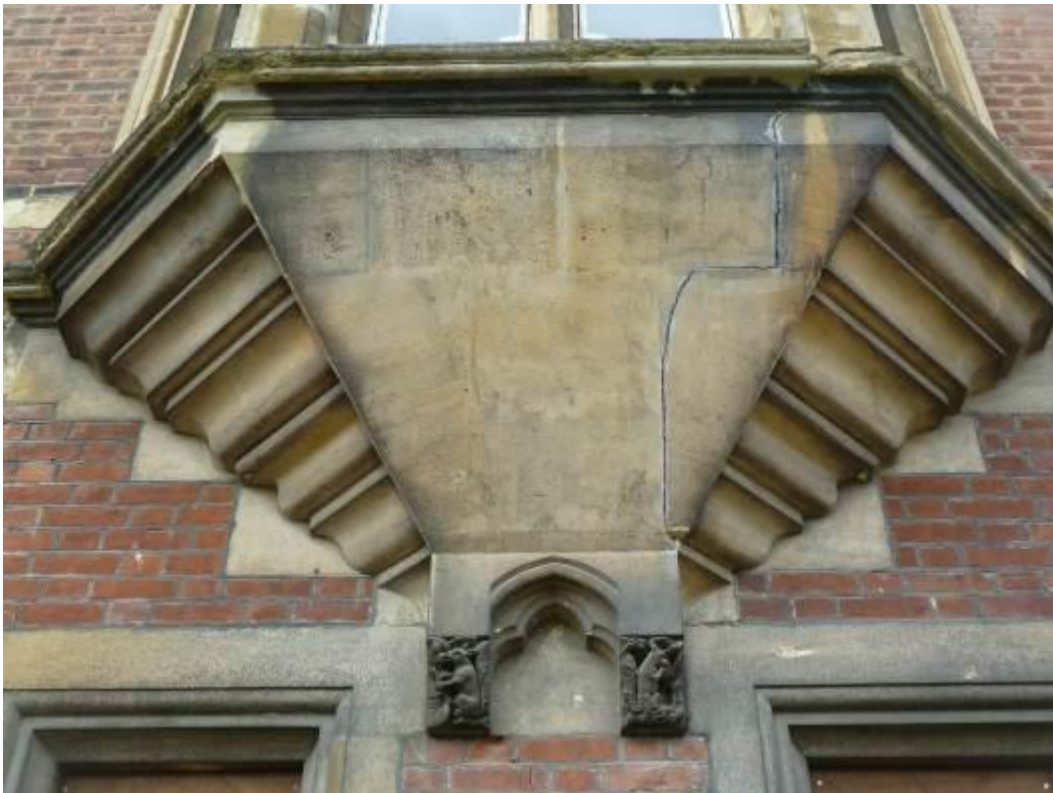
MMP50 Base of oriel window on north elevation with carved animals (March 2016)
