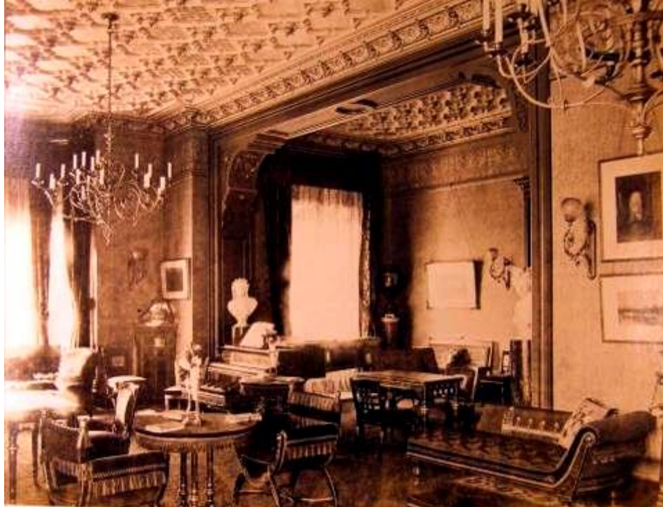
MMJ8 080179/8 shows the Drawing Room looking into the recess. This was later blocked. All the decorative features, including the elaborate cornice, and cusped panelled ceiling, with mini pendants, were swept away in a 1920s redecoration.
