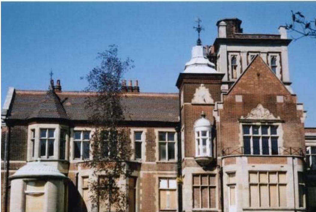
MMP3, 4 South Elevation in 2007 showing simplified gable and turret. The railings around the bay window roof at right are simplified substitutes.
