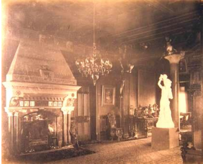
MMJ6. 080179/7 shows the Hall, looking across from the staircase recess. The hooded fireplace, panelled Drawing Room door, pilaster, polished Granite column and heavy beamed ceiling were all removed in a later remodelling. The corbel blocks are glimpsed.
