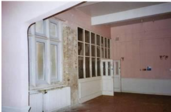
MMP18, 19 Simplified (1920s) screen in Entrance Hall and Tudor Arch on landing
