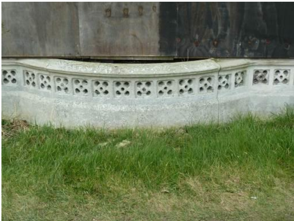
MMP52 Fretted stone planter at base of outer face of porte cochere (March 2016)
