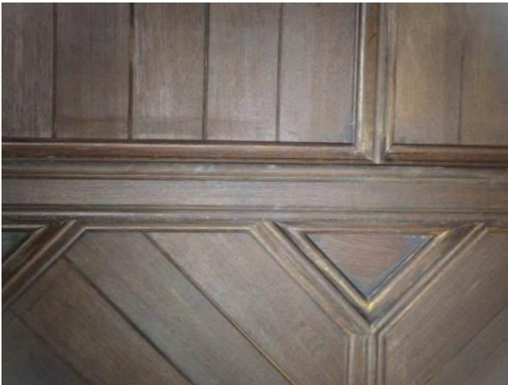
MMP 47 Original state of ceiling, preserved above later corridor (March 2016)
