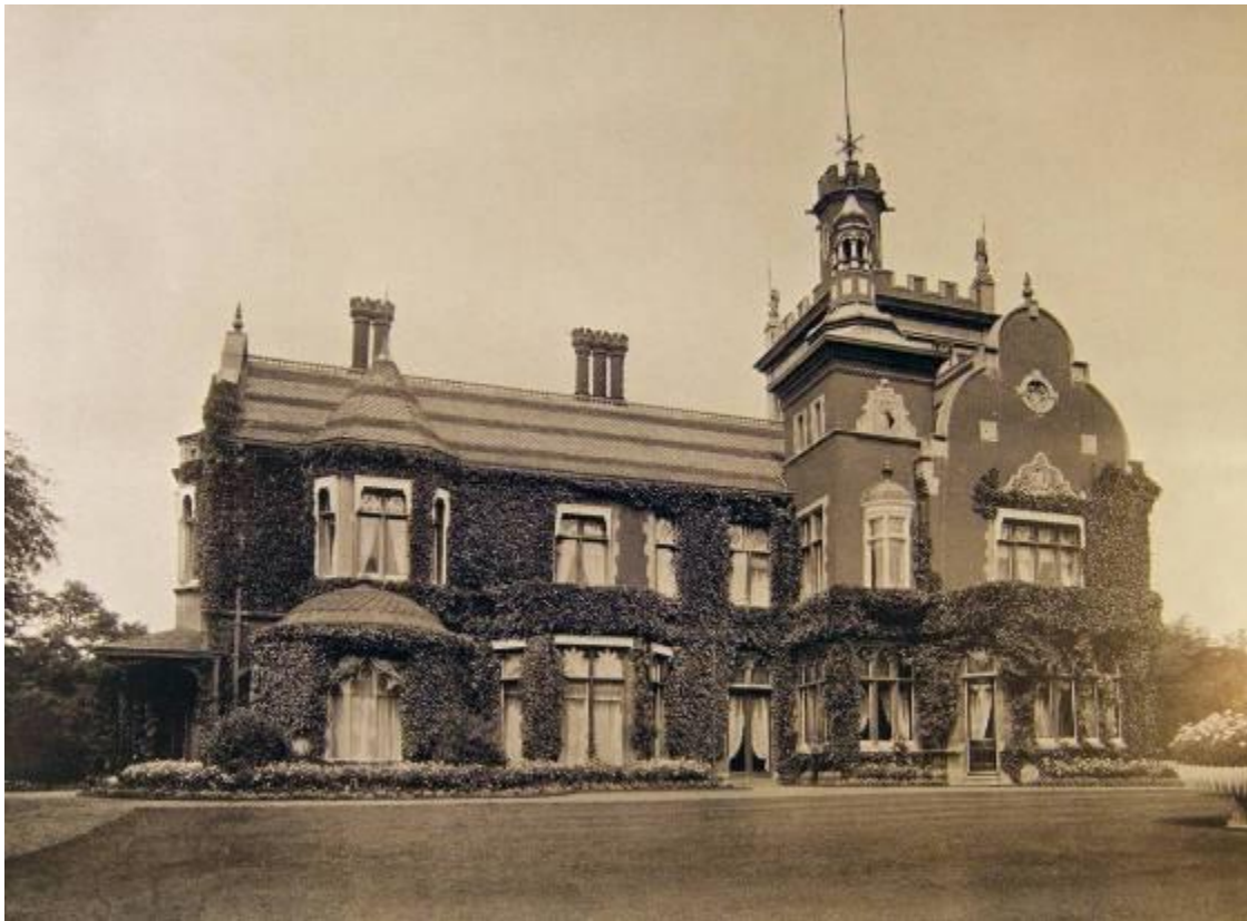
MMM4. South front showing circular pavilion extension at left. Ivy obscures balcony details.
