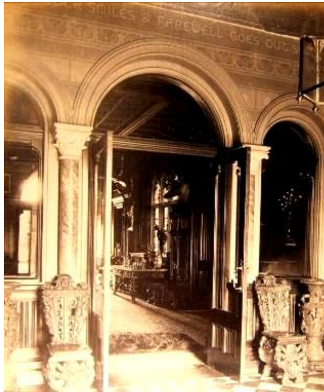
MMJ7. 080179/10 shows the ante-hall looking into the main hall. Although the layout survives, the screen was much simplified in the 1920s. None of the decoration (somewhat in the style of Christopher Dresser) survives. All panelling of main hall was stripped – some of bracketed ceiling remains. The window looking into the inner area evidently had stained glass inserts, and cusped heads.
