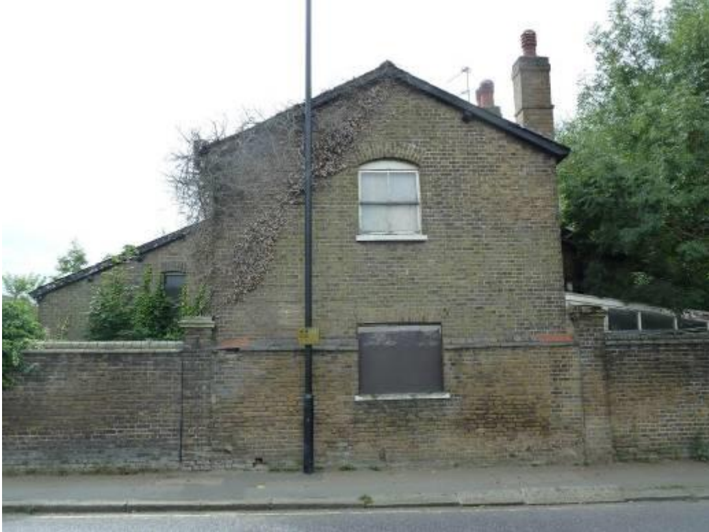
MMP35 North elevation of Caen Cottage above boundary wall: the various additions all predate 1948.
