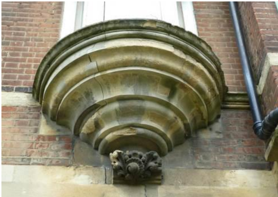
MMP54 Carved boss at base of cupola tower south elevation (March 2016)
