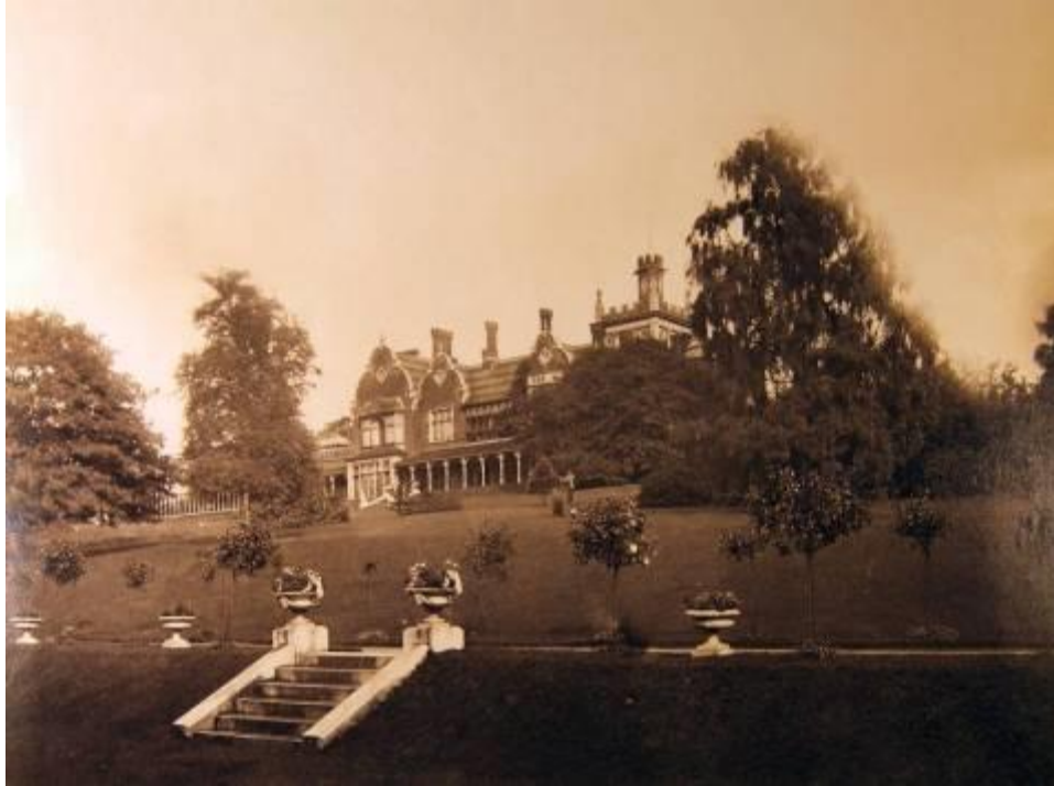
MMJ4. 0800179/5 This view shows the house from the lower garden, looking towards the west elevation. Much of the detail of the south corner and return elevation is obscured by trees. However, it can be seen that there were projecting gargoyles below the crenellations of the upper stair turret above parapet level of the tower, and that heraldic beasts bearing flag standards stood on the square corner plinths of the tower parapet. The pierced stonework parapet above the right hand canted first floor bay is visible. The elaborate detail of the shafted chimneys is visible in a generalised way. The pent rooflight of the picture gallery is just visible above its crenellated parapet. Other details are as described above.
