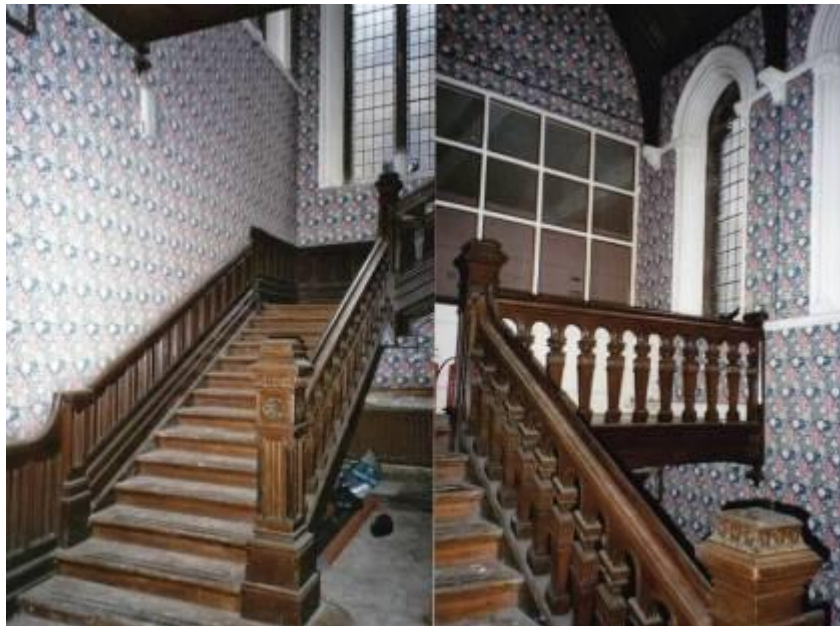
MMP20, 21 Detail of staircase, the major intact historic internal feature
