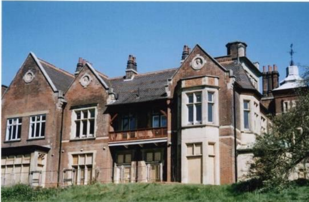
MMP5,6. Turning from the South to the West Elevation, the surviving group of full height chimneys are clearly visible behind the cupola roof on the lower photograph
