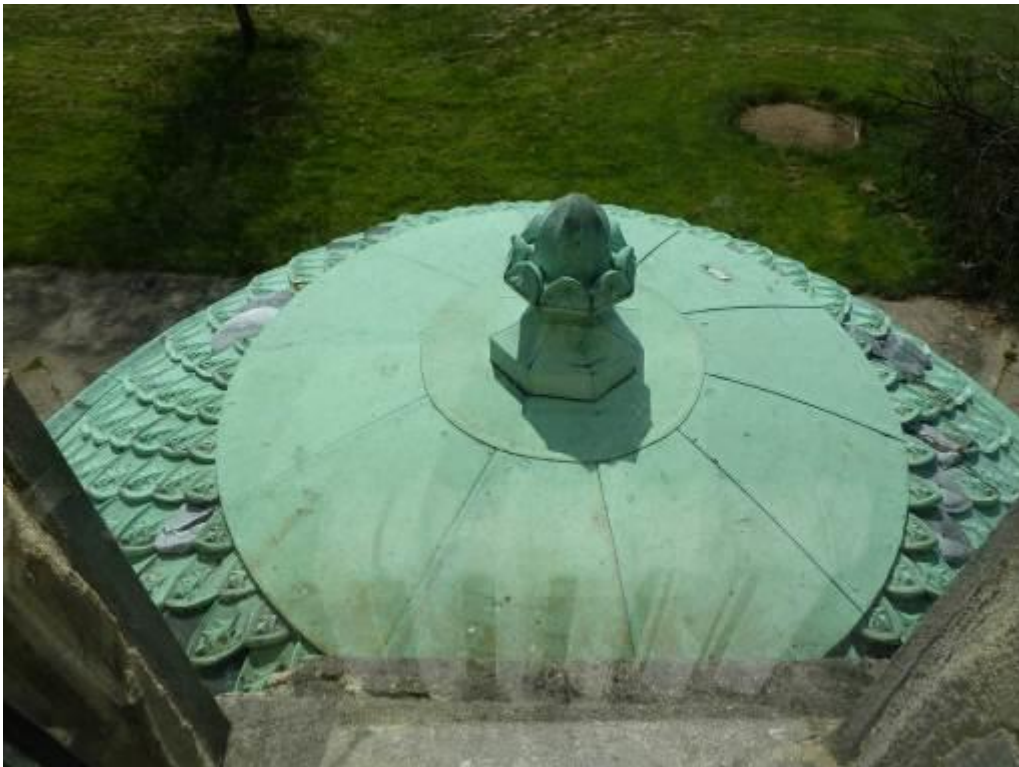
MMP45 Detail of copper roof of pavilion (August 2014)
