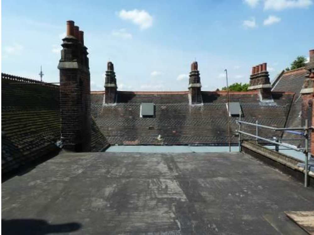
MMP41 Post 1948 reconstructed flat roof over landing (August 2014)
