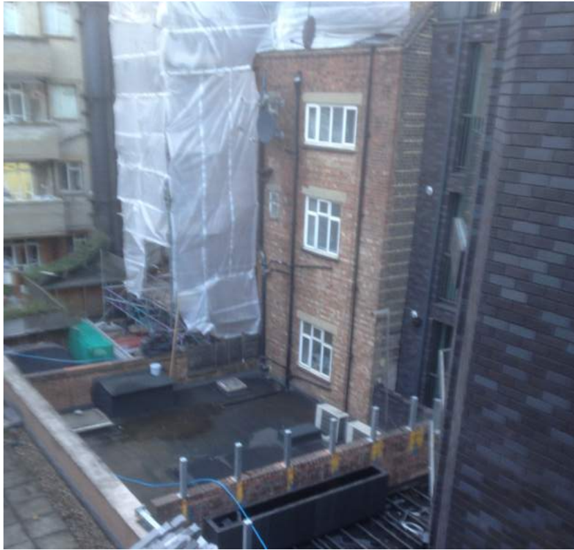
Photograph of rear of 9 Goodge Street showing adjacent properties
