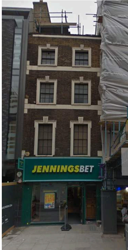
Photograph of front of 9 Goodge Street
