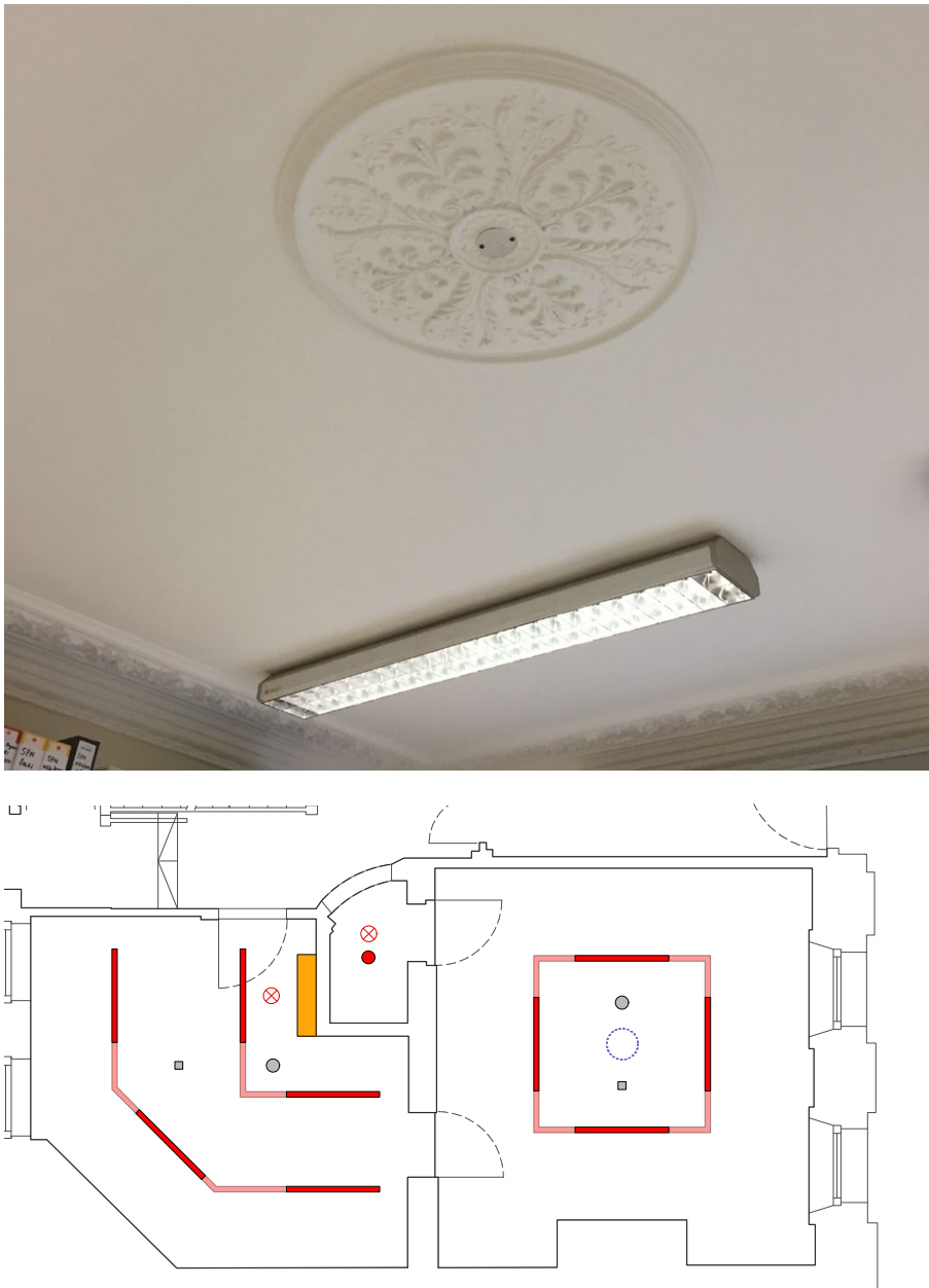
02. Existing plastered ceiling and rose within Office 01 (G03), to be retained. The existing lighting in Office 01 and 02 is to be replaced, with suspended luminaires. Smoke detectors will be renewed in existing locations. Please refer to Appendix for details on existing and proposed lighting layouts.
