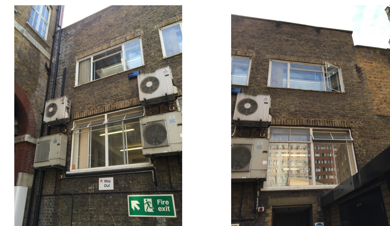
Site photos of existing wall-mounted condenser units on North facade.
