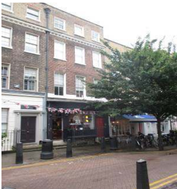
Frame No: 01 Location: Flat 3, 37 Lambs Conduit Street Description: Front Elevation Date: June 2016
