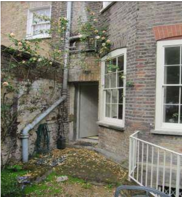
Frame No: 04 Location: Flat 3, 37 Lambs Conduit Street Description: Rear Elevation Date: June 2016
