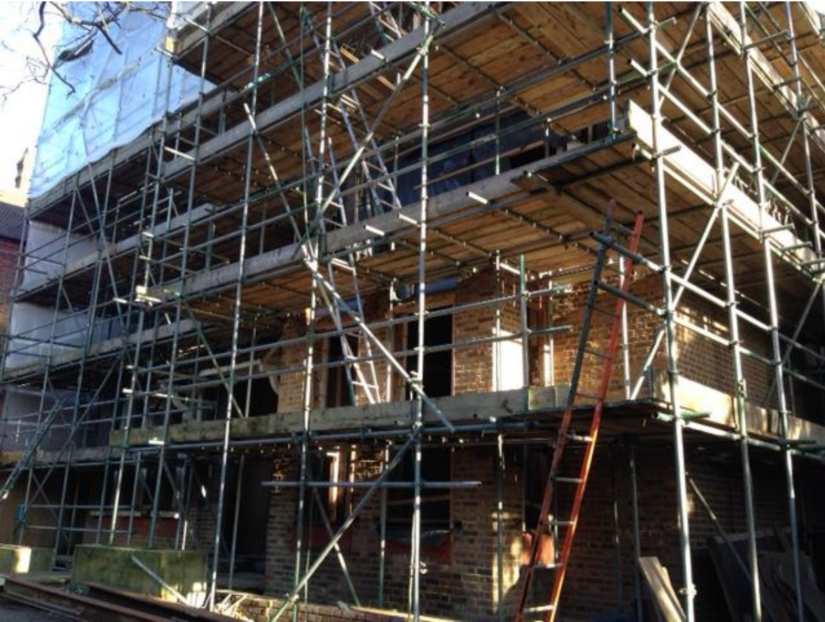
3. View towards front bay window
