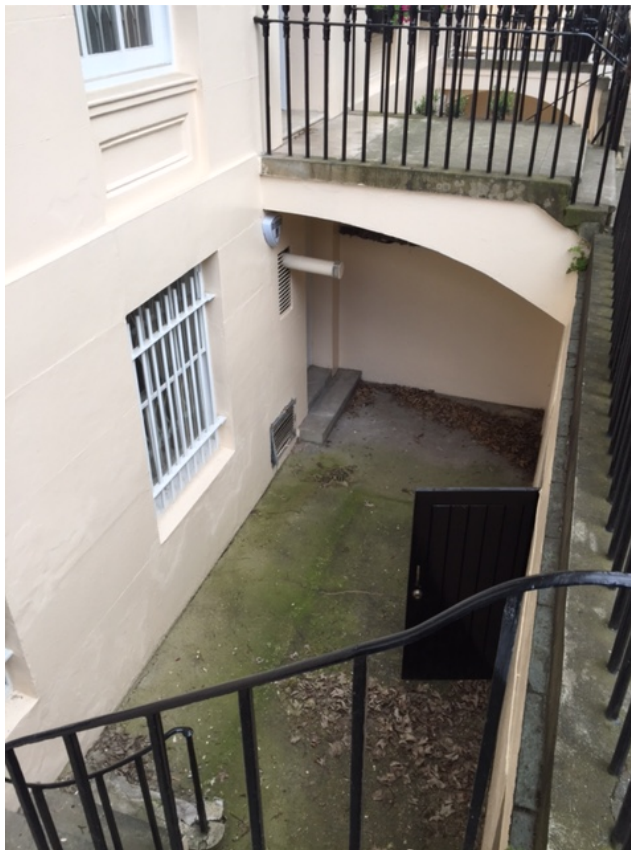
Photo 4: Front lightwell view 1
