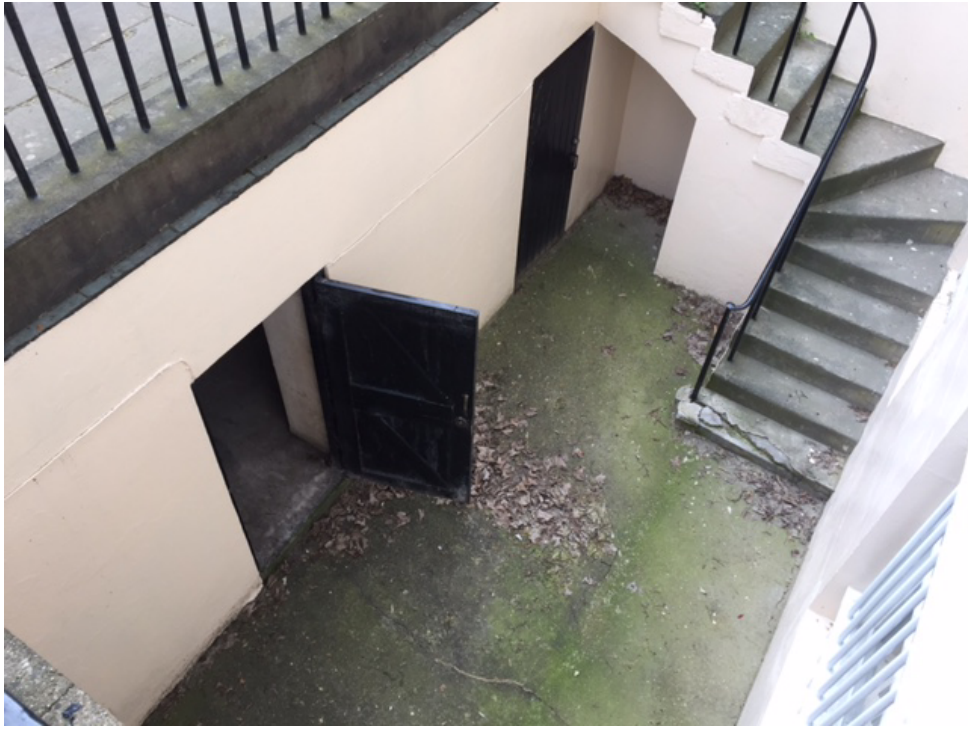
Photo 5: Front lightwell view 2
