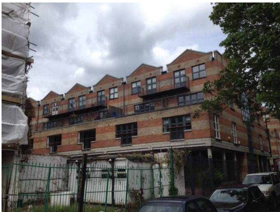
View of a rear of site Bruges Place
