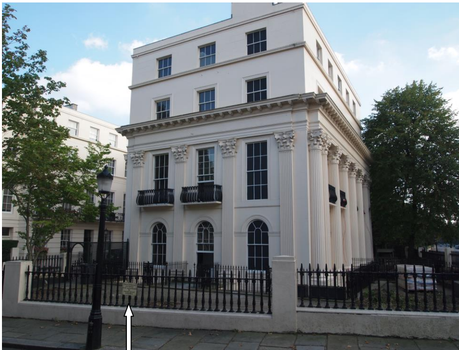
Existing warning notice
