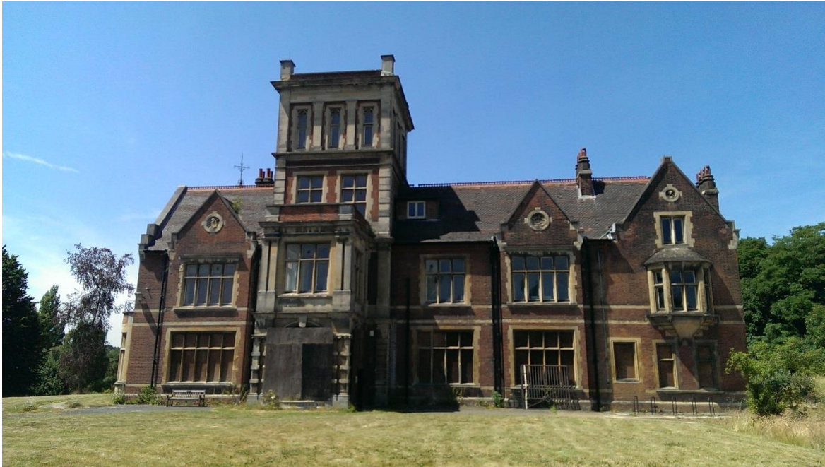
Figure 2 East View of Existing Building
