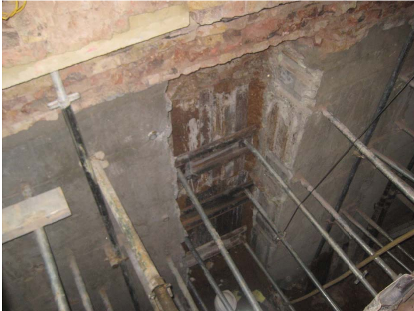
Figure 6 Example of trench sheet back propping
