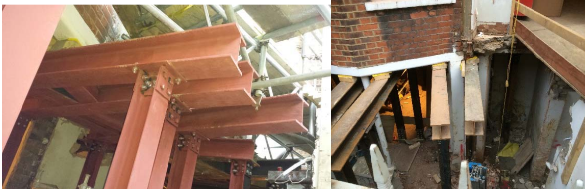
Figure 1 Example of needling to existing wall
