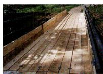
Ground Protection GP2 - Option 2 - For more permanent small plant and pedestrian movements ground protection in the form of a single thickness of scaffold boarding supported by scaffold, as opposite, can be adopted to oridge areas and avoid compaction.
