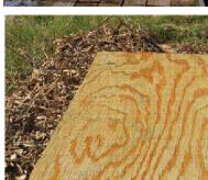
Ground Protection GP3 - For Pedestrian movements ground protection in the form of a single thickness of scaffold boards or plywood on top of a compressible layer (Woodchip) laid onto a geotextile, or supported can be used to form the access or provide a sub base to other ground protection.
