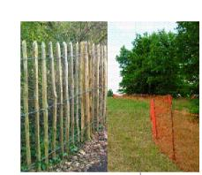
Type 3 Tree Protection Fencing (TPF3) This is to be erected as a visual barrier to protect areas designated for no or later construction. Consisting either stock fencing, post and rail fencing, Chestnut Pale fencing or Orange Extruded Plastic
