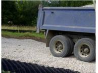
**No Dig-Ground Protection GP1 -** Option 2 For high use areas or were heavy vehicles are expected, substitute traditional dig out and compacted stone infill with an above ground **Cellweb** or similar, to avoid the need for excavation and limit compaction – may be retained as a porous sub base for hard Surfacing within the scheme.
