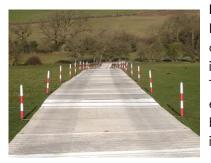
**No Dig-Ground Protection GP1 -** Option 1 For lower traffic areas, where heavy vehicles are expected, substitute compacted stone infill with a temporary above ground Trackway. This avoids the need for excavation and limits the weight of material build up and limits compaction when installed with compressible sub-surface.
