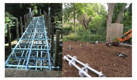
**Example 2 – Thrust or Bored Piles**. Small plant piles can be installed within Root protection area. To enable heavy buildings to be supported several smaller piles can be connected to form a pile cap providing improved support as shown below.
