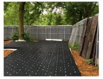
No Dig-Ground Protection GP1 - Option 3 Void forming system such as Permavoid or ArborRaft act as a protection to the tree roots and avoid the need for excavation. These systems also limit the weight of material build up and can be installed with compressible sub-surface. – may be retained as a porous sub base for hard surfacing within the scheme.
