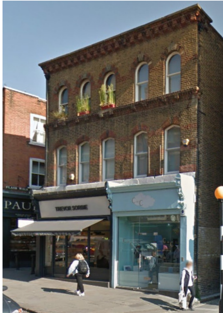
No. 41-42 Hampstead High Street
