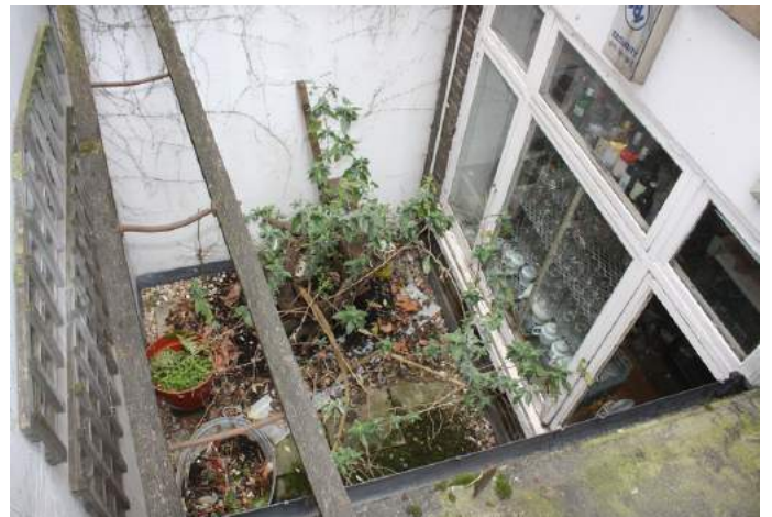
Interior of Cafe, basement room and rear yard.
