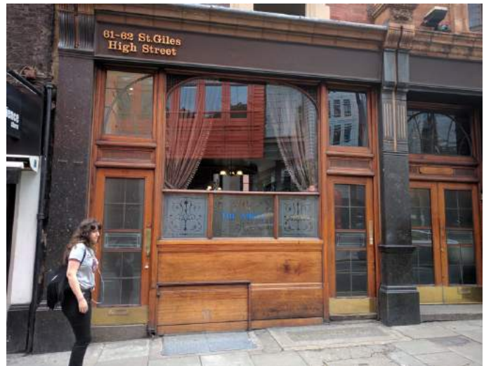
Timber framed cafe bar elevation on St Giles High Street within frame of pilasters and entablature.
