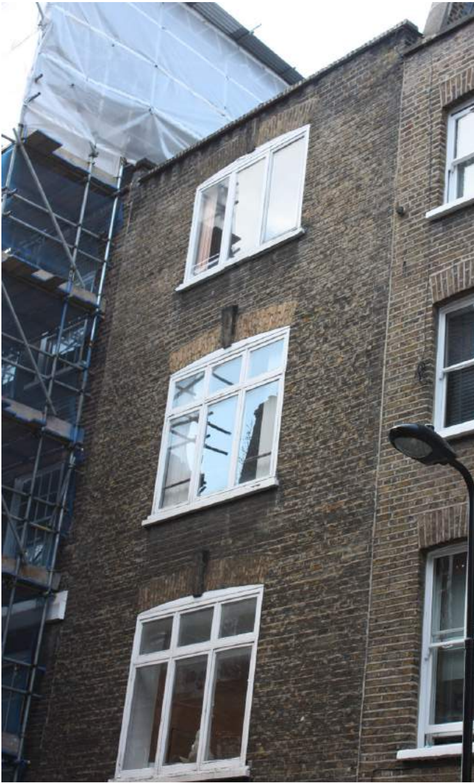
Windows on Betterton Street above Cafe, note rotten timber sill sitting on original stone sill.
