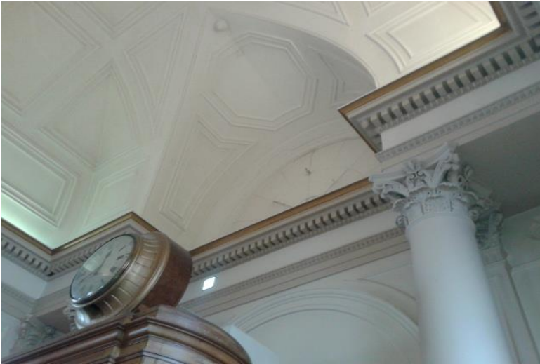
124355 Hairline fractures in library ceiling
