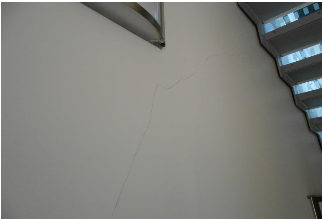
1428 Fracture to wall within stairwell
