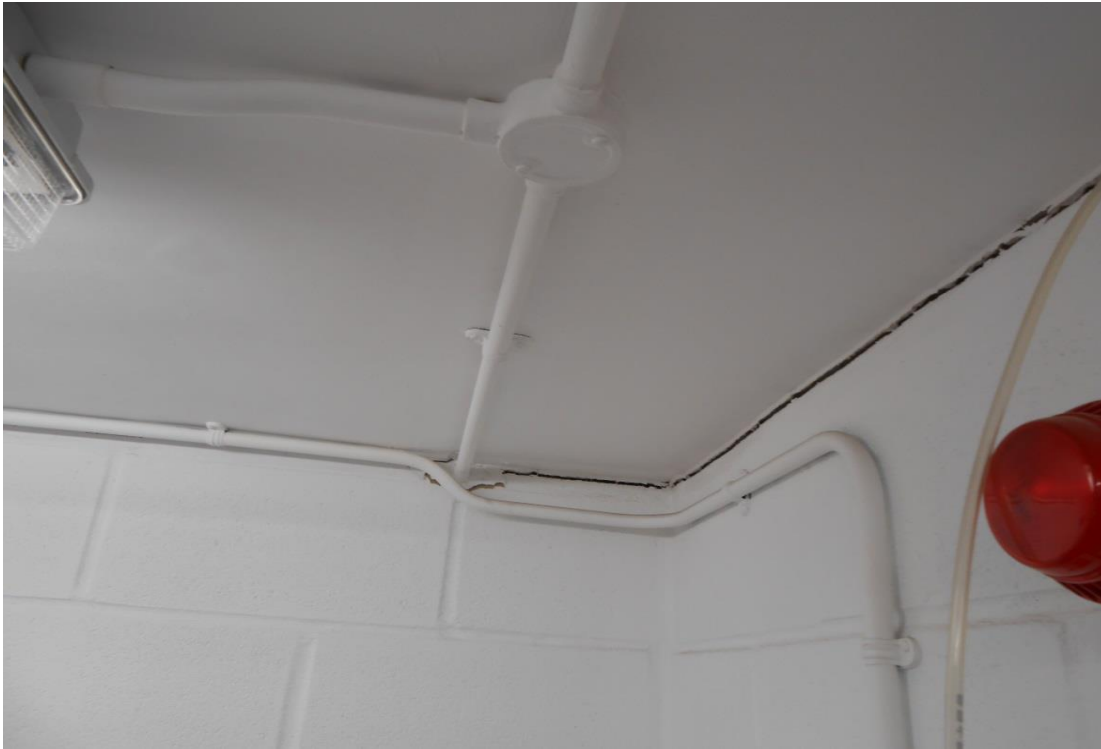
1577 Fracture - at high level which runs from Room 2.10 - 2.12A
