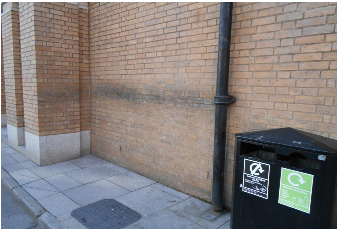
Staining to brick work on formal entrance
