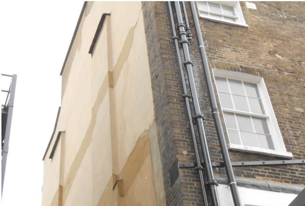
Side and rear elevation showing further patch repairs and tie bars
