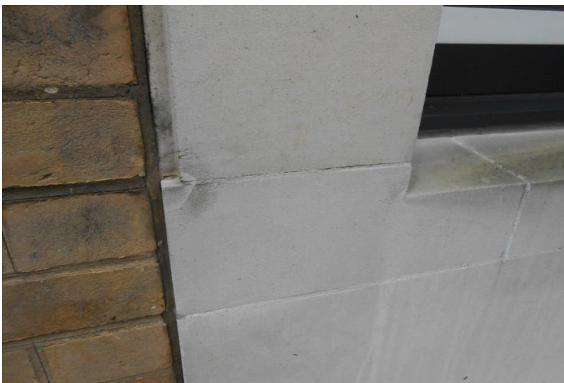
Damage and staining to stone surrounds
