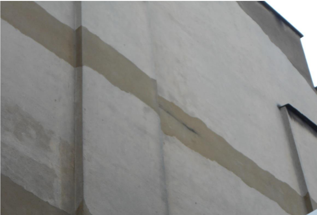
Side elevation, with previous patch repairs and further cracks
