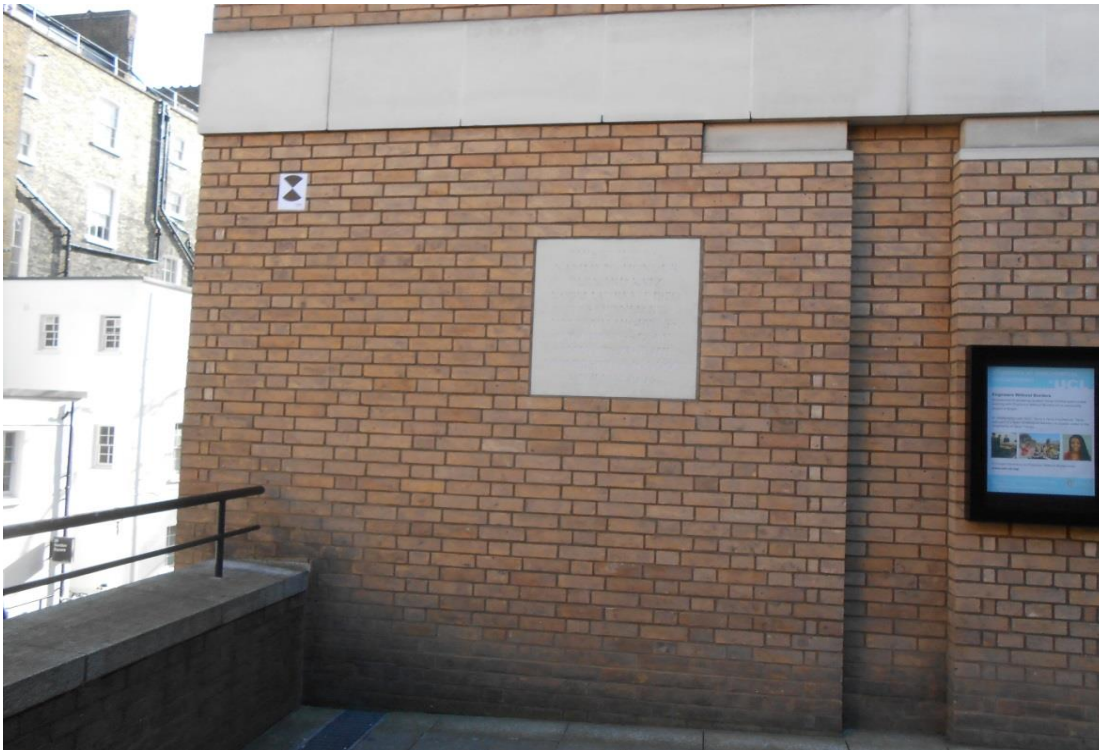
Japanese Garden elevation showing staining to brick work at low level and inset stone plaqu
