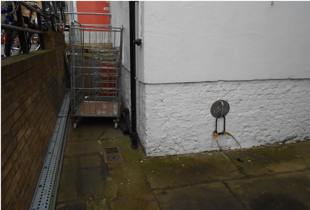
Rear of outshot - painted brick work at low level, with render finish
