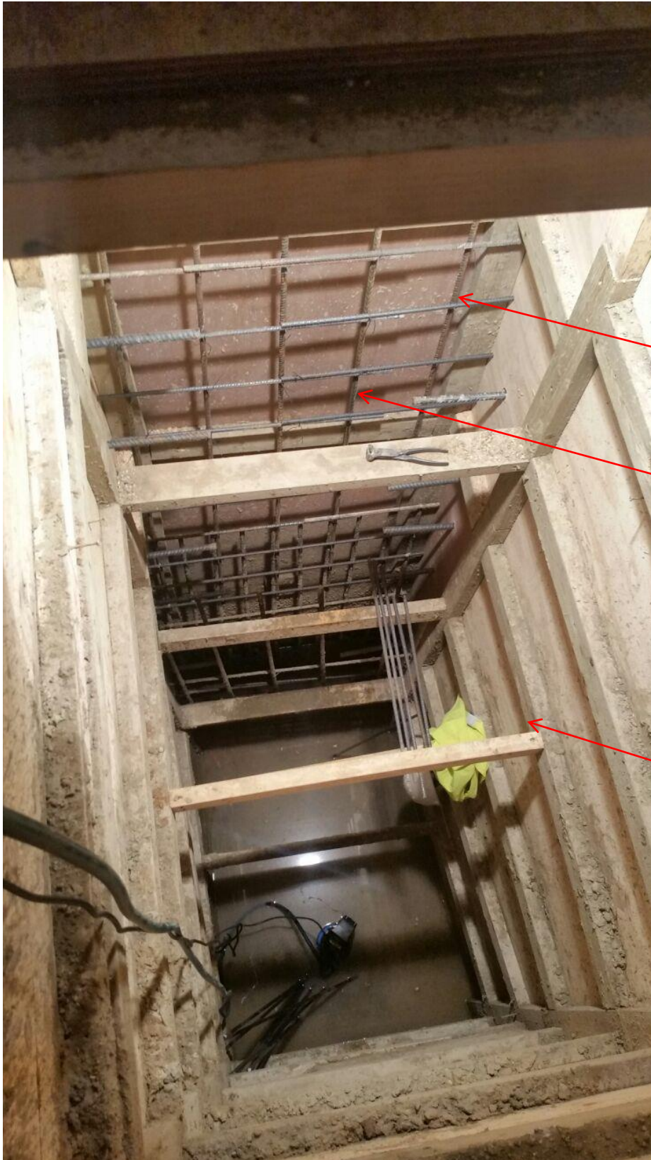
Photo 1- Typical Pin Access Pit (View from top down)
