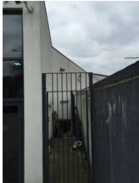
Edge of building on northern aspect.
