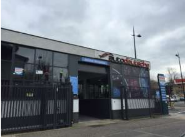
South-western aspect of the building
