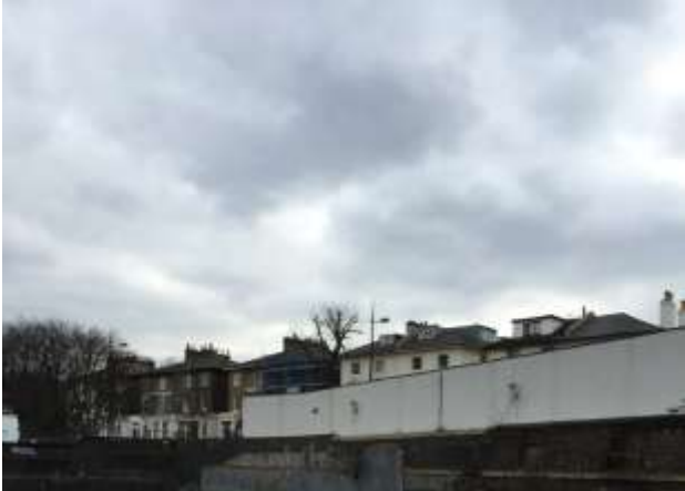
Northern aspect of the building. Viewed from a distance.
