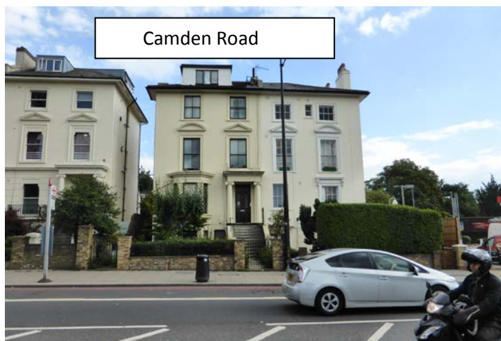
Figure 4 - Residential Flats Camden Road opposite proposed site (No.208-212)
