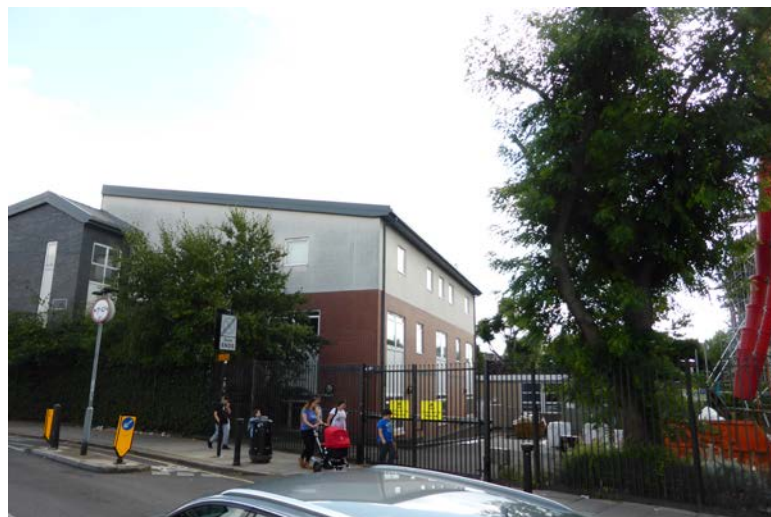
Figure 6 - Girls School Building (B1) on Sandal Road near Camden Road. (windows NW facing )
