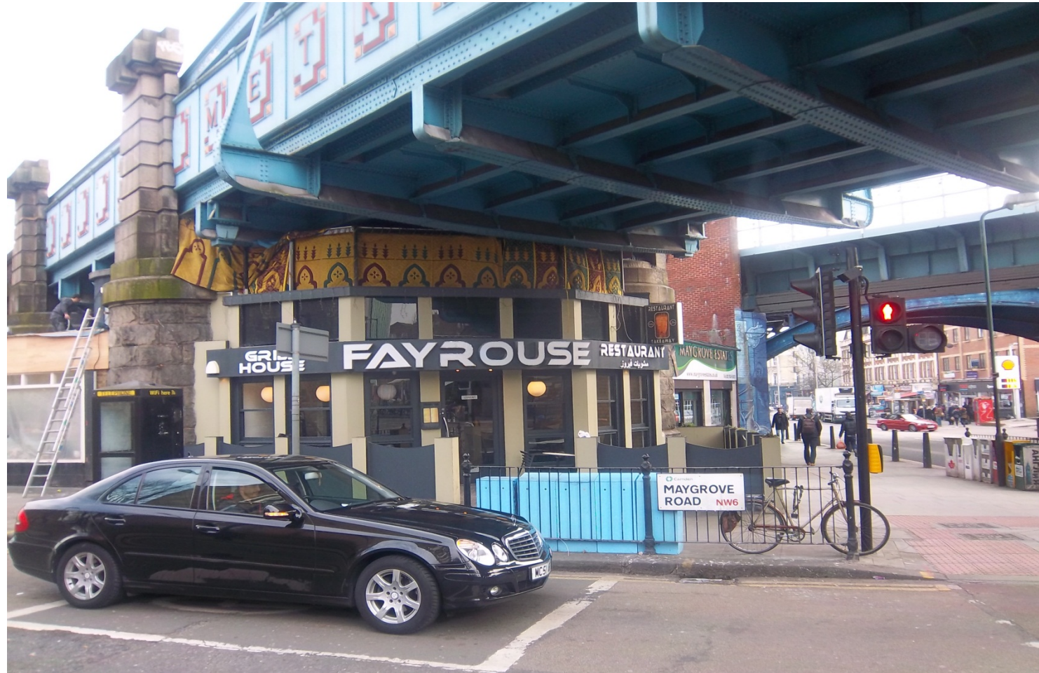
Existing restaurant (A3) on junction of Maygrove Road and Kilburn High Road
