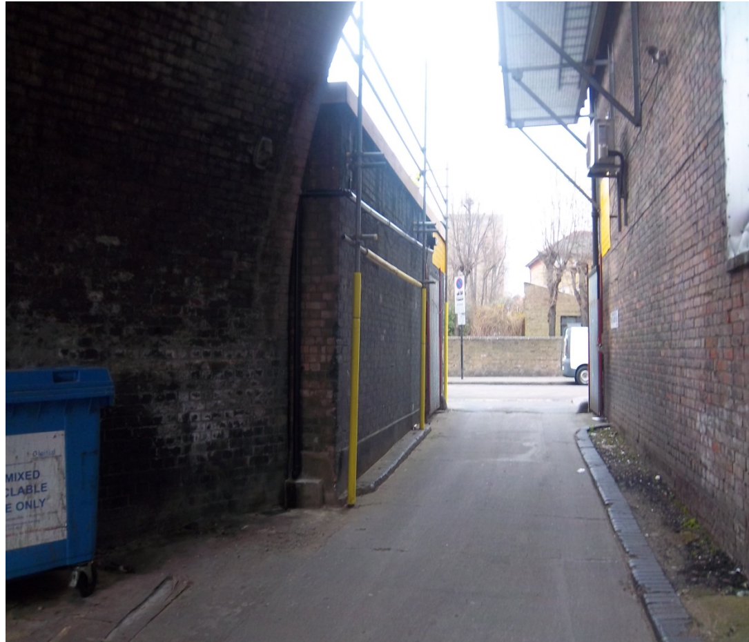
Access way to garages and side elevation of application property
