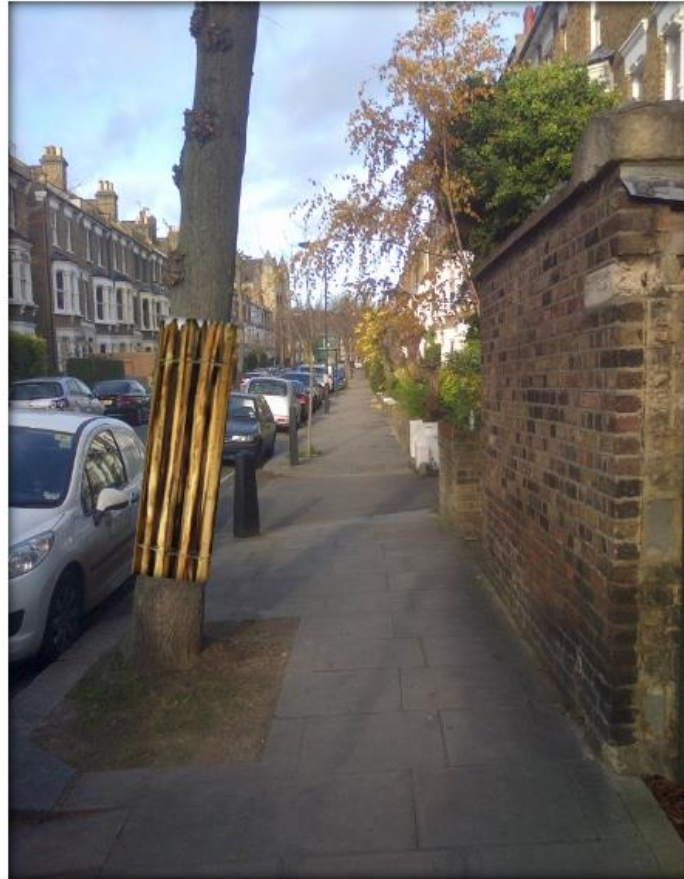
Figure 1: showing the 'chestnut pale fencing' to be applied to tree T01 – Common Lime
