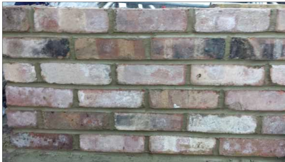
2 Facing Brick Sample Panel Photo 2 N.T.S.
