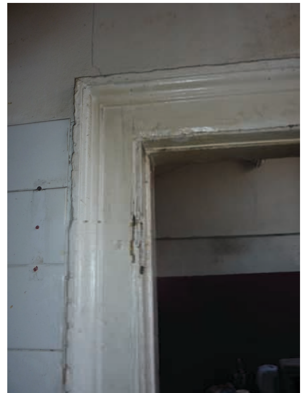
5 Photo of Existing Door Frame 1F N.T.S.
