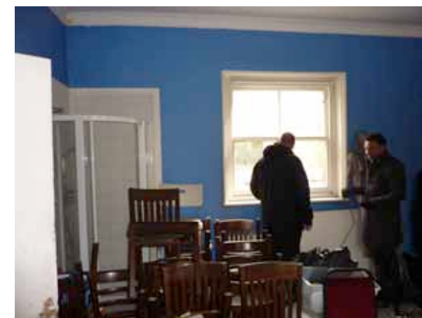
Rear Window (South Elevation)
