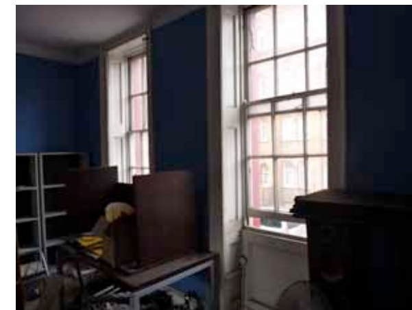
Front Window (North Elevation)
