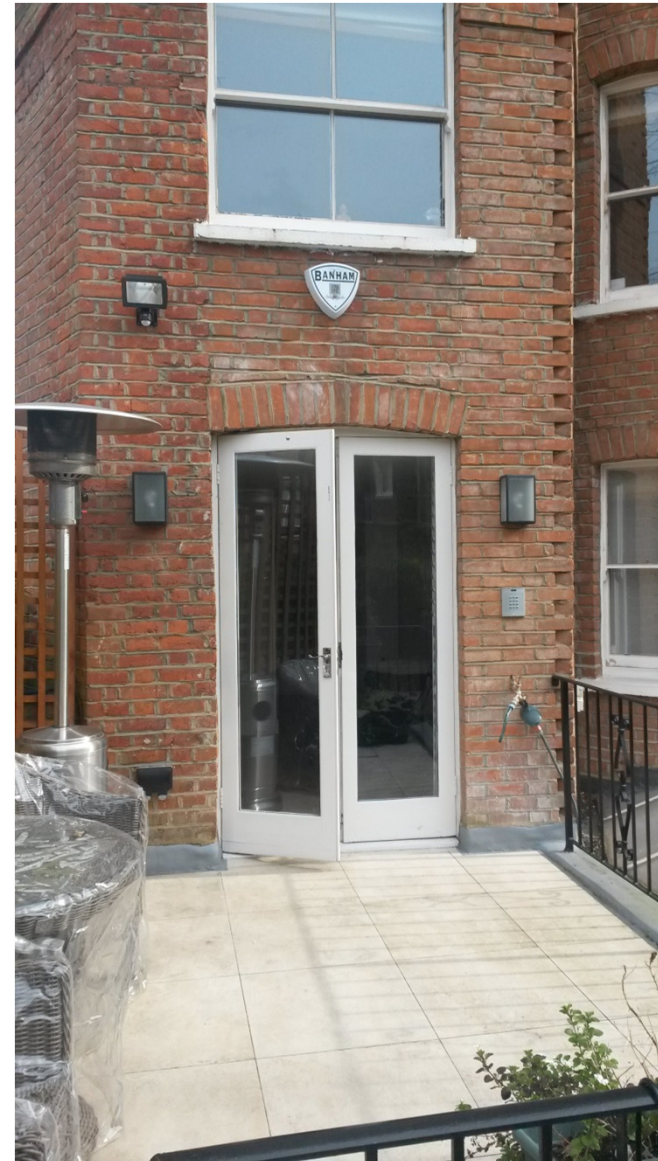
Figure 4: Existing patio doors will be retained.
