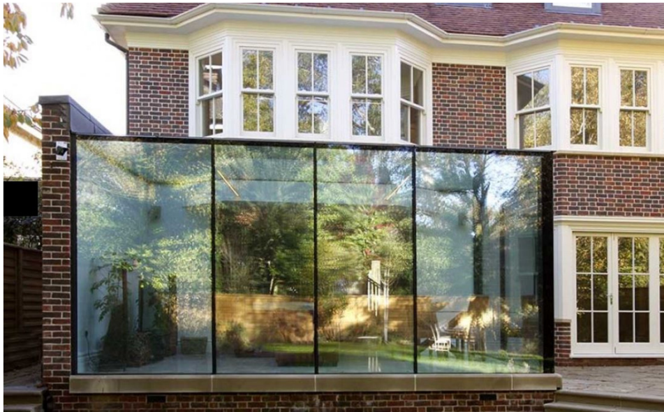
Figure 5: Example full brick wall, part brick part glazed wall design. The pre chosen manufacture has constructed in the past.
