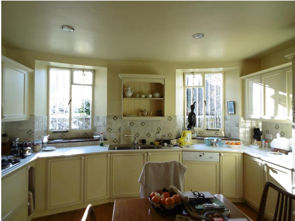
Figure 3.6: Kitchen to rear room of lower ground floor, showing metal casement windows
