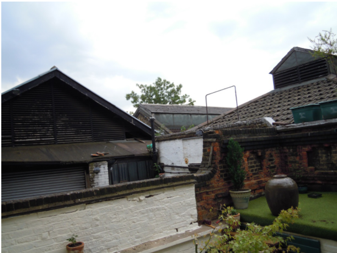
View of roofs from adjoining flat
