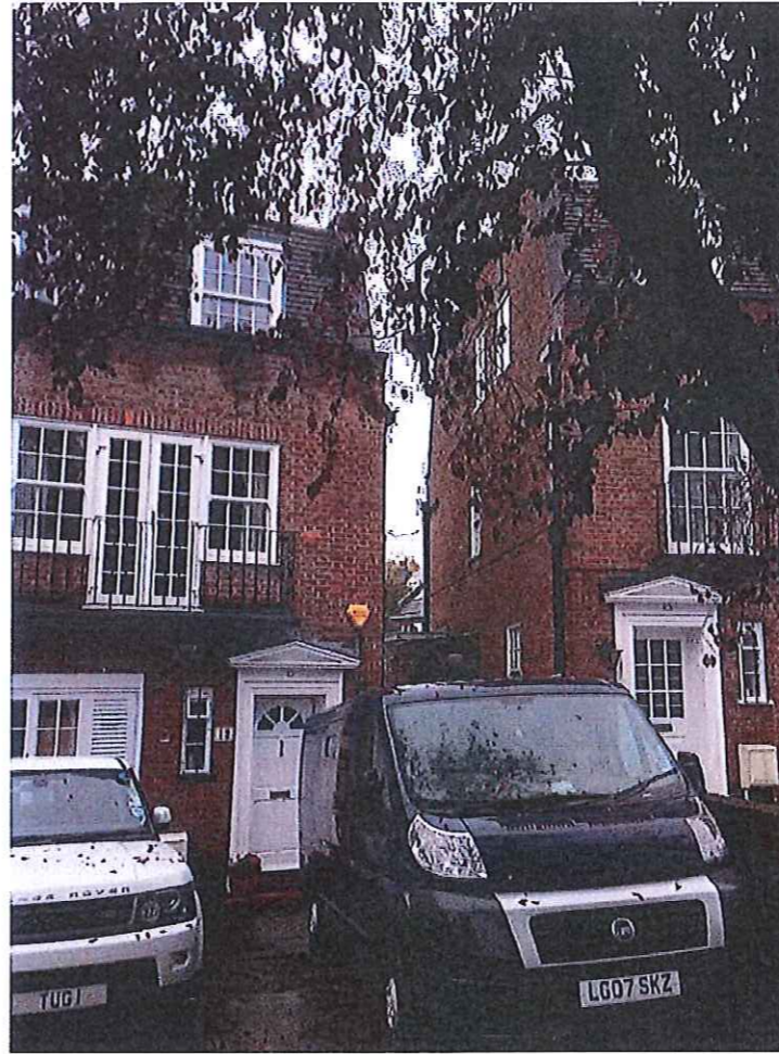
FRONT VIEW (No.12 on the left & No.10 on the right.)
