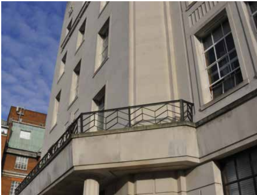
Detail of Bentham House exterior
