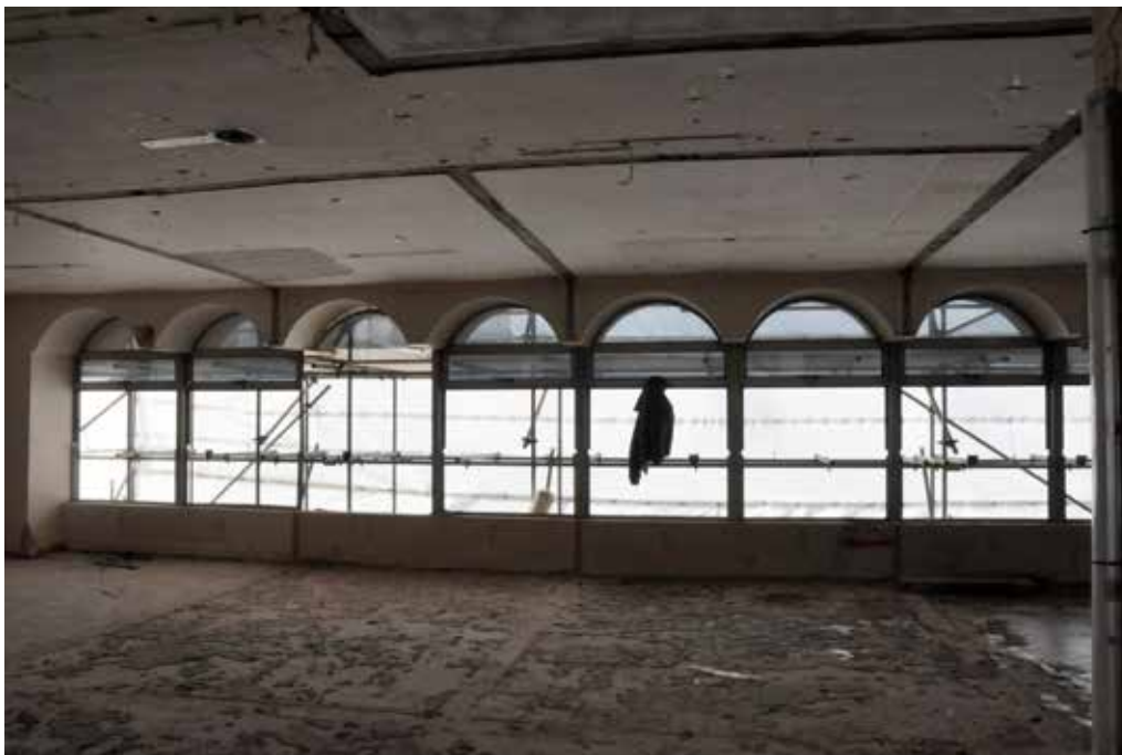
Interior of Gideon Schreier Wing: first floor interior stripped out in 2016
