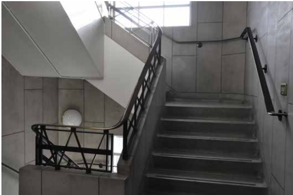
Staircase in north-east corner
