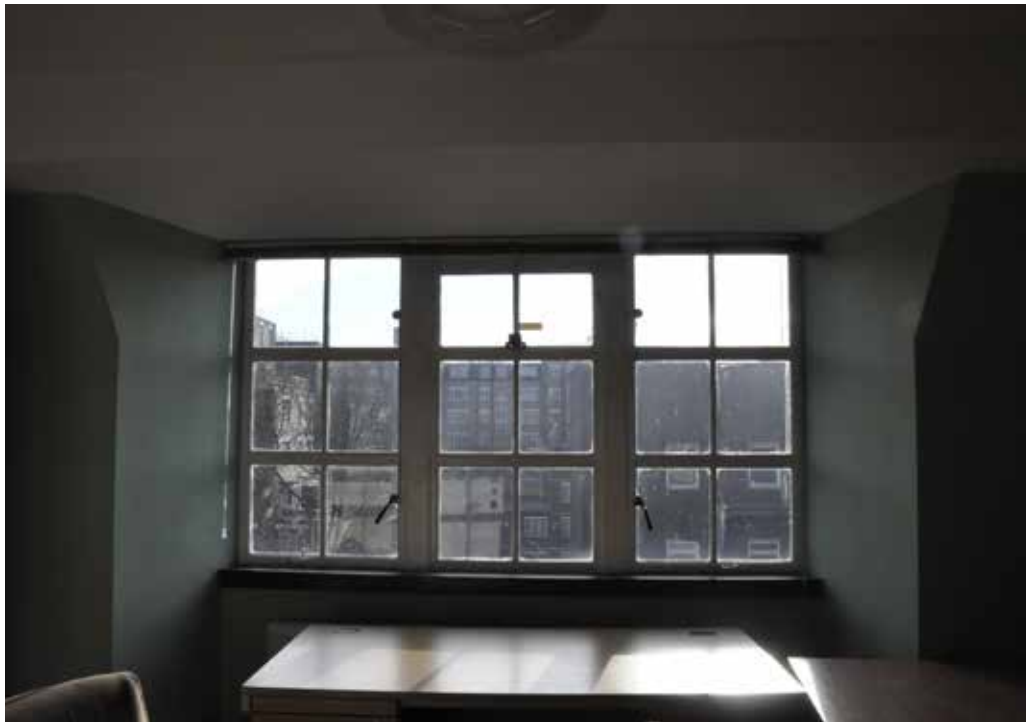
Windows on the fifth floor of Bentham House
