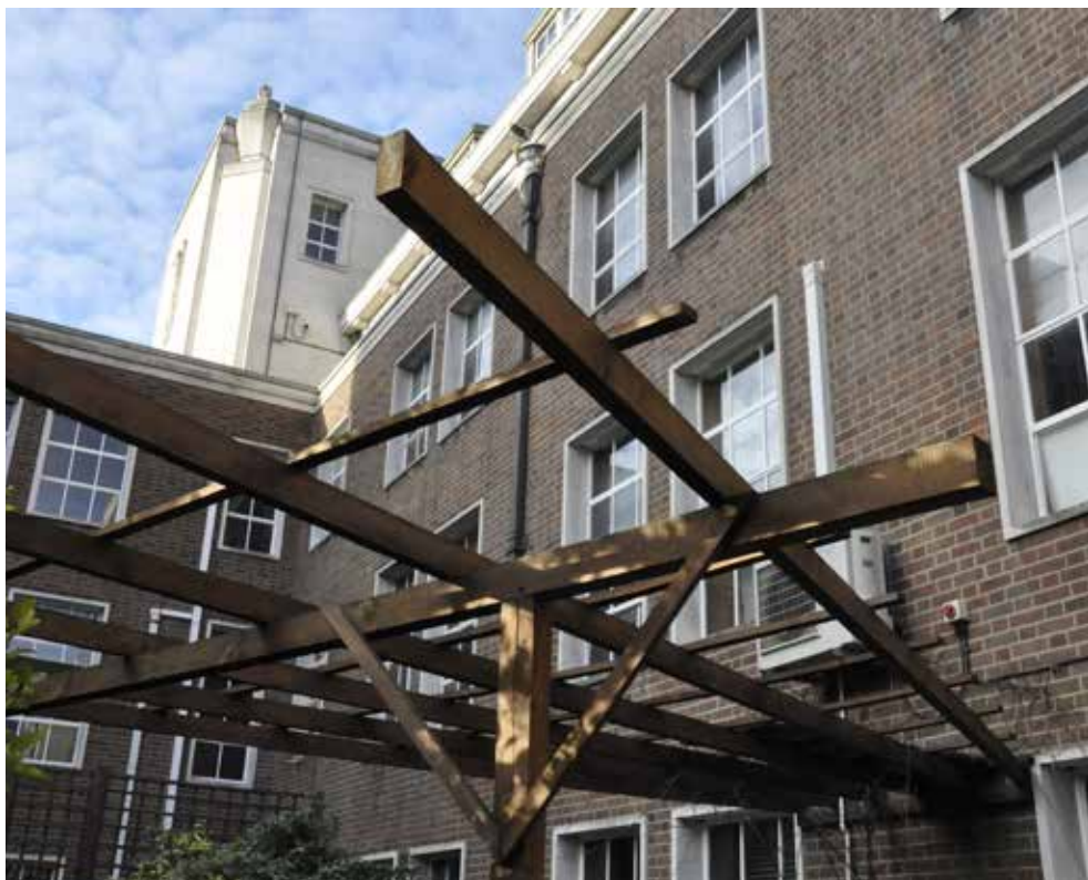
Bentham House rear elevation
