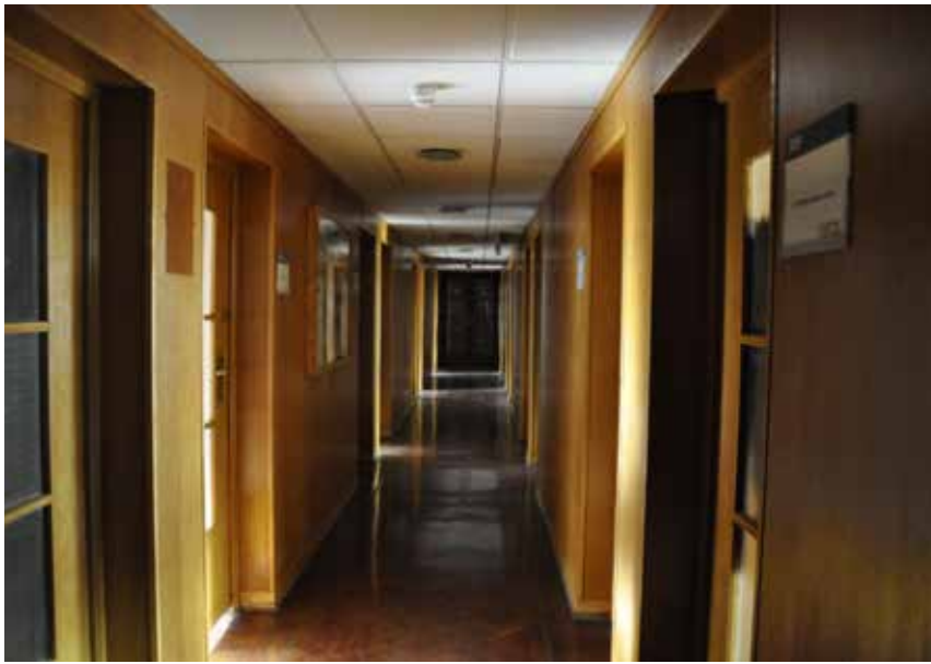
Timber panelling on third floor corridor of Bentham House
