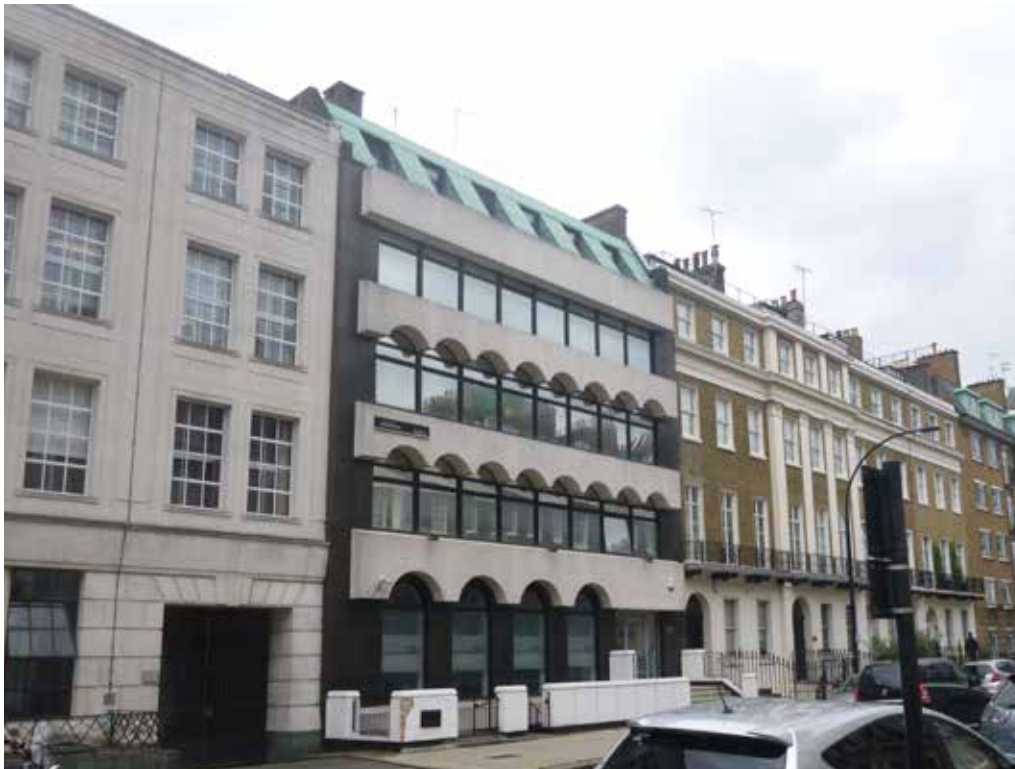
Gideon Schreier Wing before the start of building works (2014)
