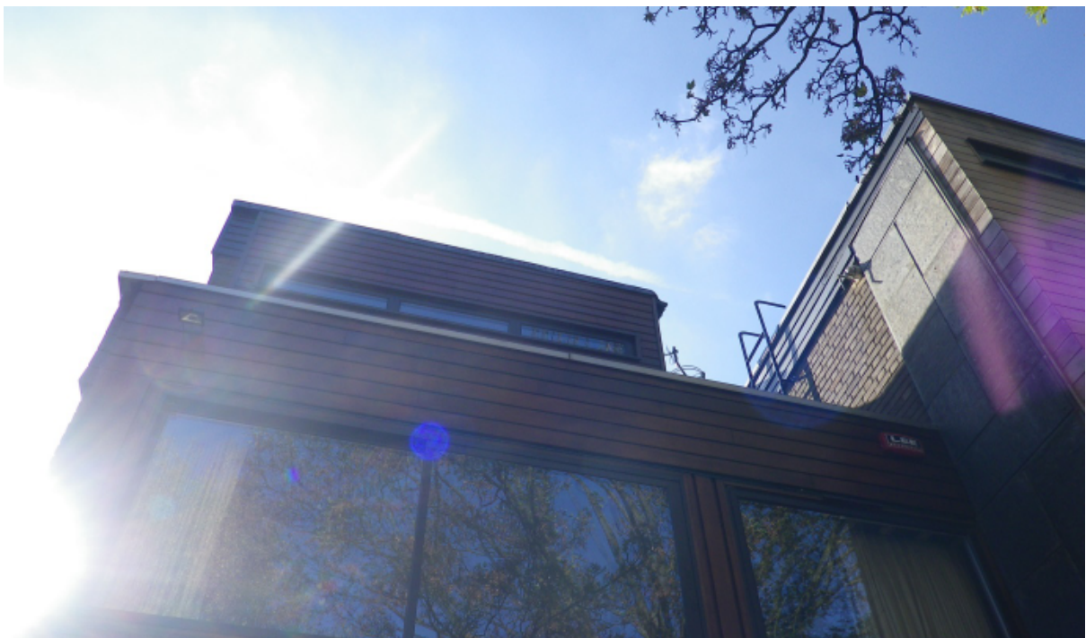
Roof of nos. 7 and 8 Oak Hill Park Mews
