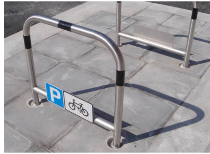
3 N° secure cycle spaces provided using 'Sheffield' style security bars imbedded in the existing conc. floor finish
