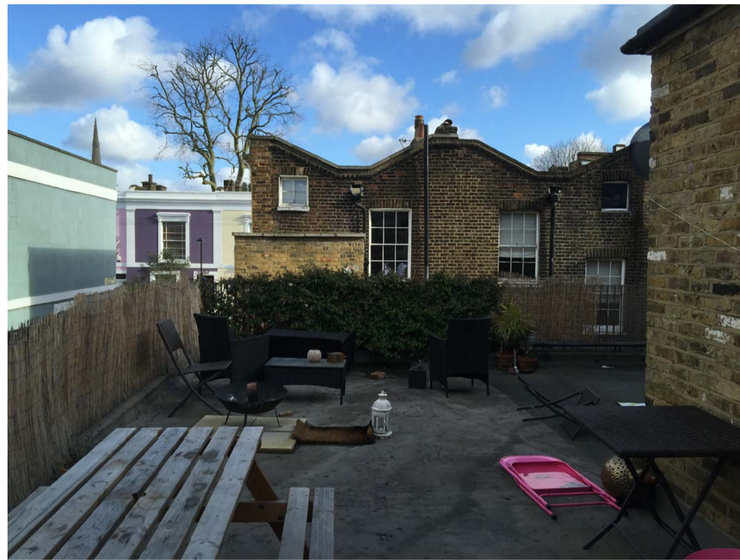
EXISTING TERRACE LOOKING EAST
