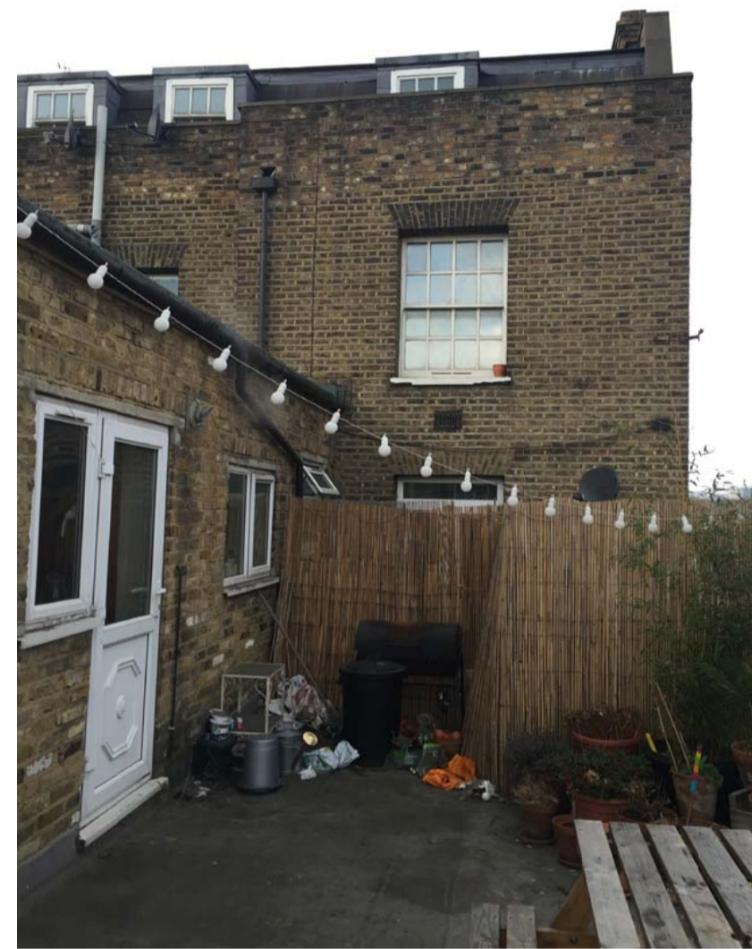
EXISTING TERRACE AND EXTERNAL DOOR
