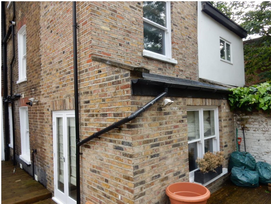
Photograph 3 – Existing Rear Extension
