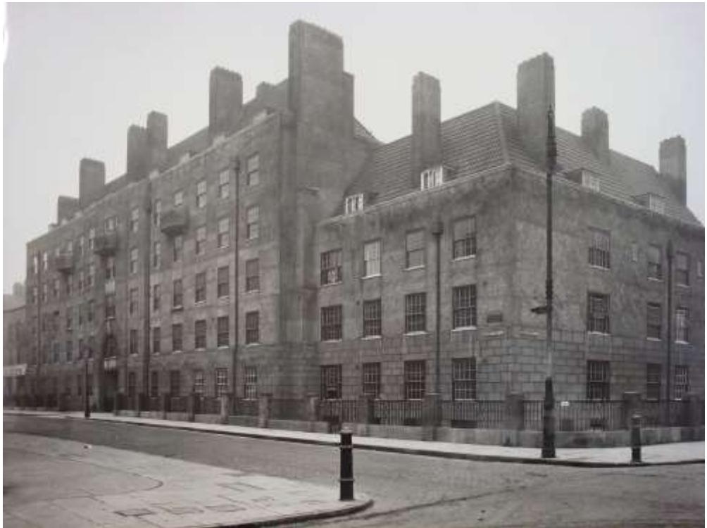
Figure 10: Walker House, Southern Block/Phoenix Street Elevation, 1929
