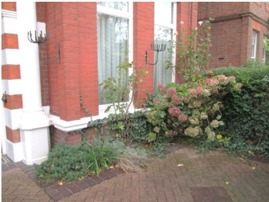
55 Lancaster Grove – ground floor windows
