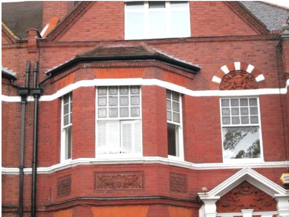
55 Lancaster Grove – first floor windows
