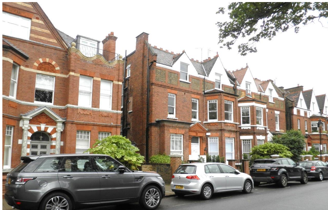
View looking East along Lancaster Grove (from no.57)
