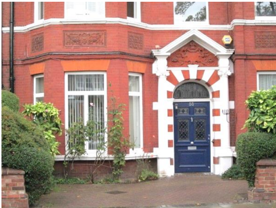
55 Lancaster Grove – ground floor bay window
