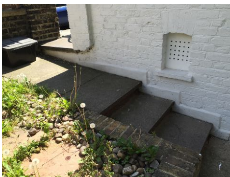
Steps down to the door of 24A
