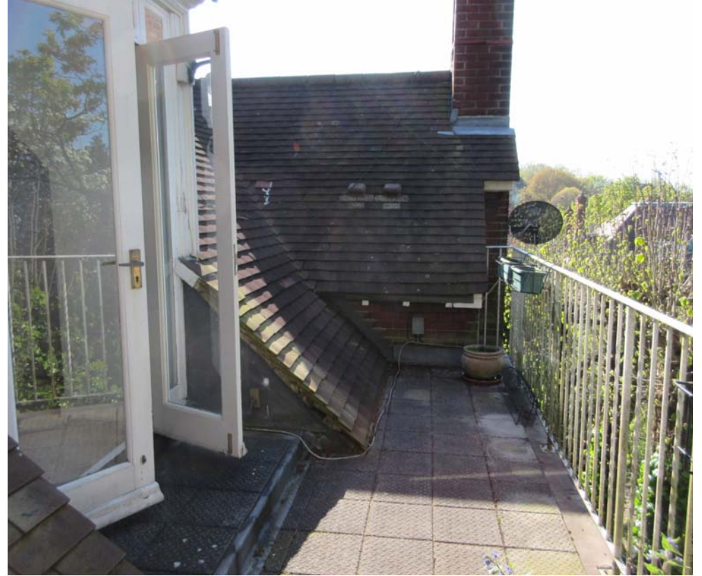
View of the existing roof terrace from the outside.
