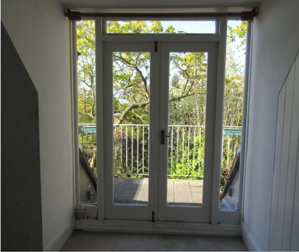
View of the existing roof terrace from the inside.
