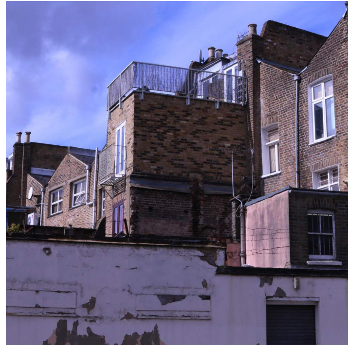
View of neighbouring extensions and roof terrace
