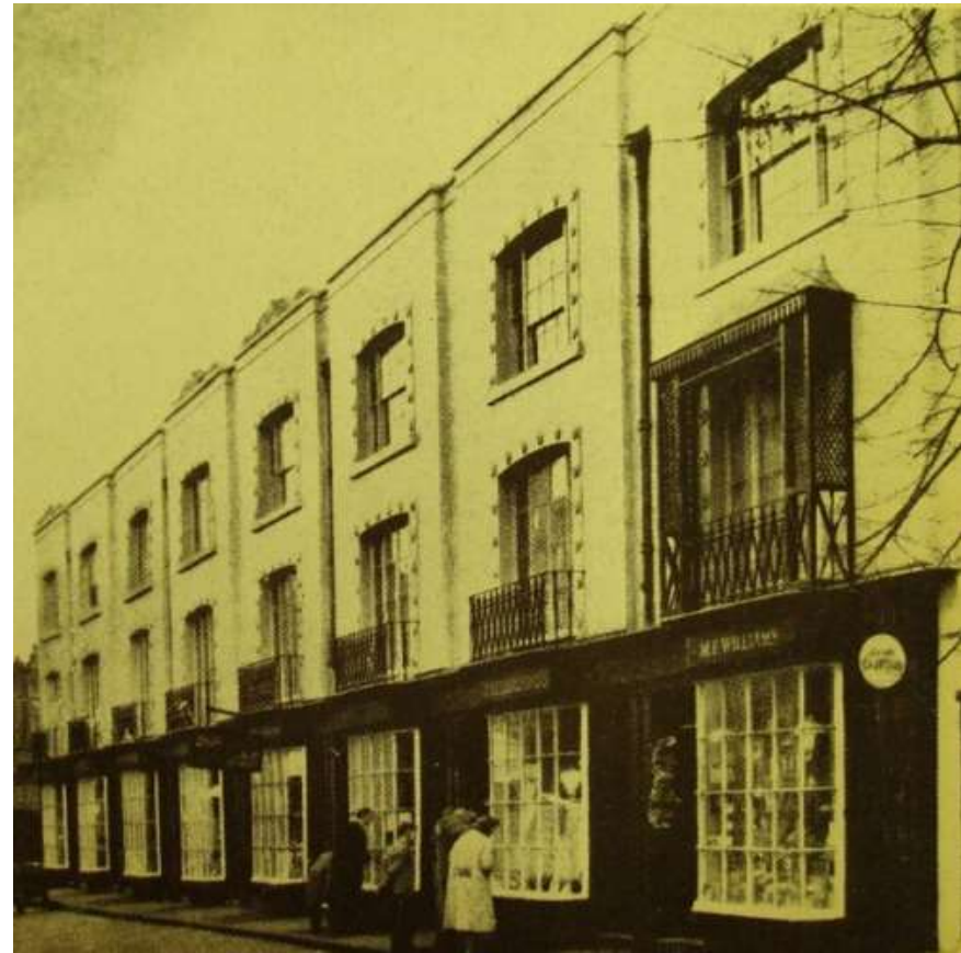
Figure 10: 1-7 Woburn Walk, Post-1961 & Restoration
